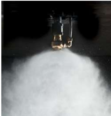
Figure 1: Two examples of hybrid water mist systems currently on the market. (left) Victaulic Vortex system discharging. (right) ANSUL Aquasonic system discharging.
