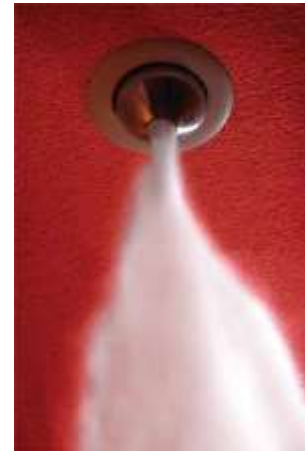
Figure 1: Two examples of hybrid water mist systems currently on the market. (left) Victaulic Vortex system discharging. (right) ANSUL Aquasonic system discharging.
