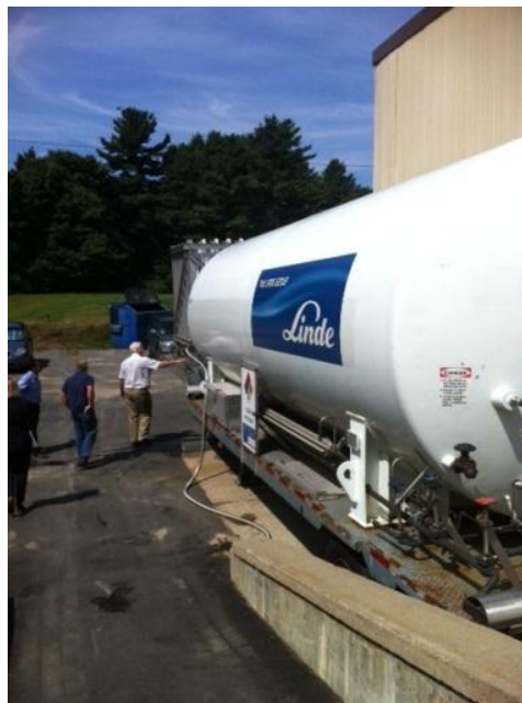
Figure 15. Nitrogen tank source of dry N_2 for the week long production of jet-milled SBC.
