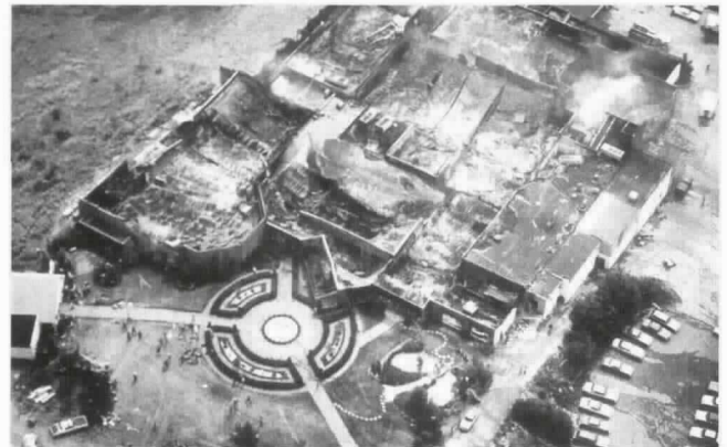
Aerial view of the Beverly Hills Supper Club fire site
