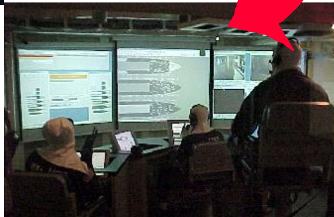
DC Central with intelligent supervisory control system aboard ex-USS Shadwell
