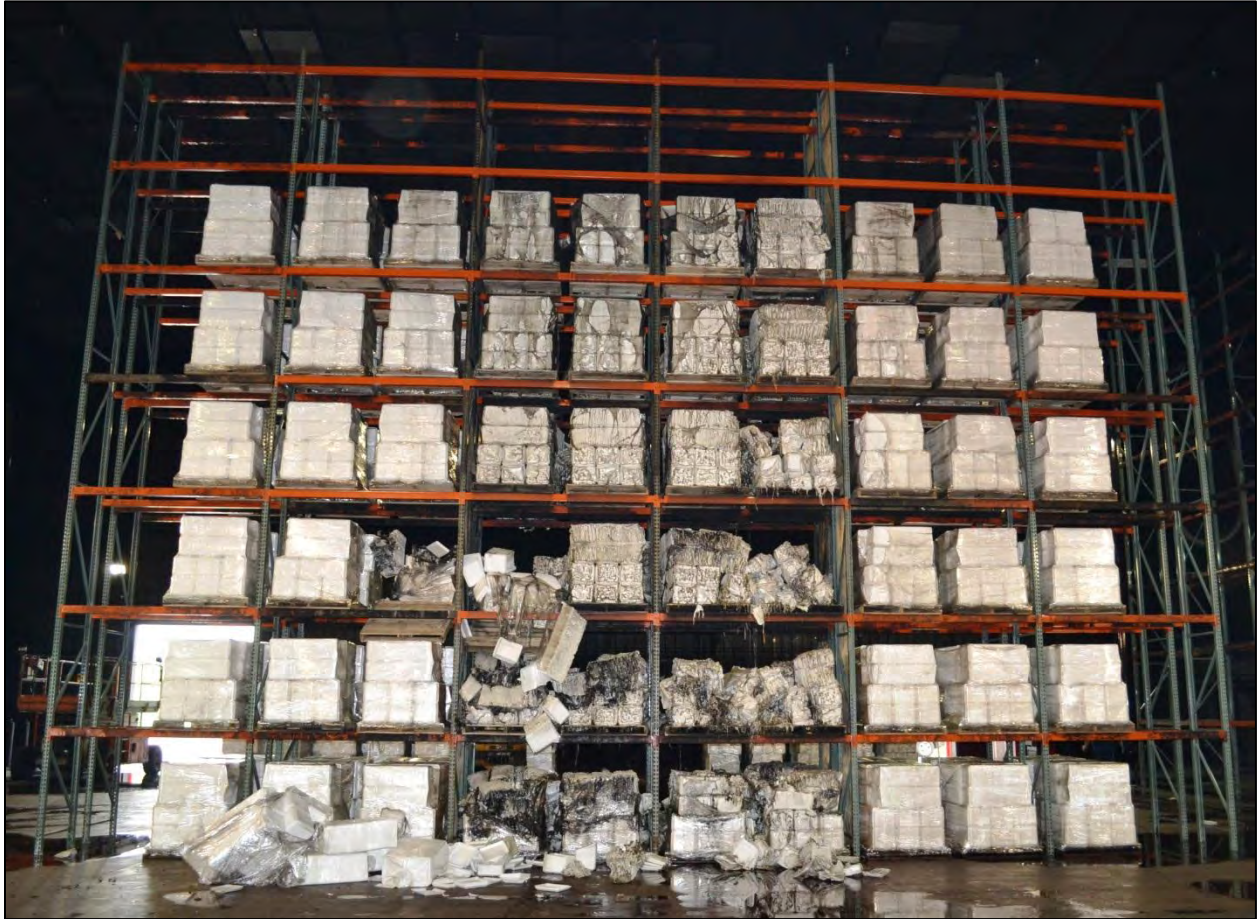
Figure B- 6 View of South Main Array
