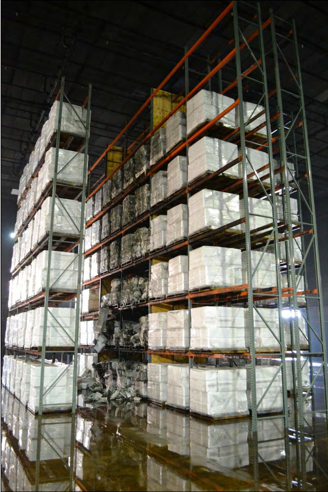
Figure B- 4 Overall View - From East
