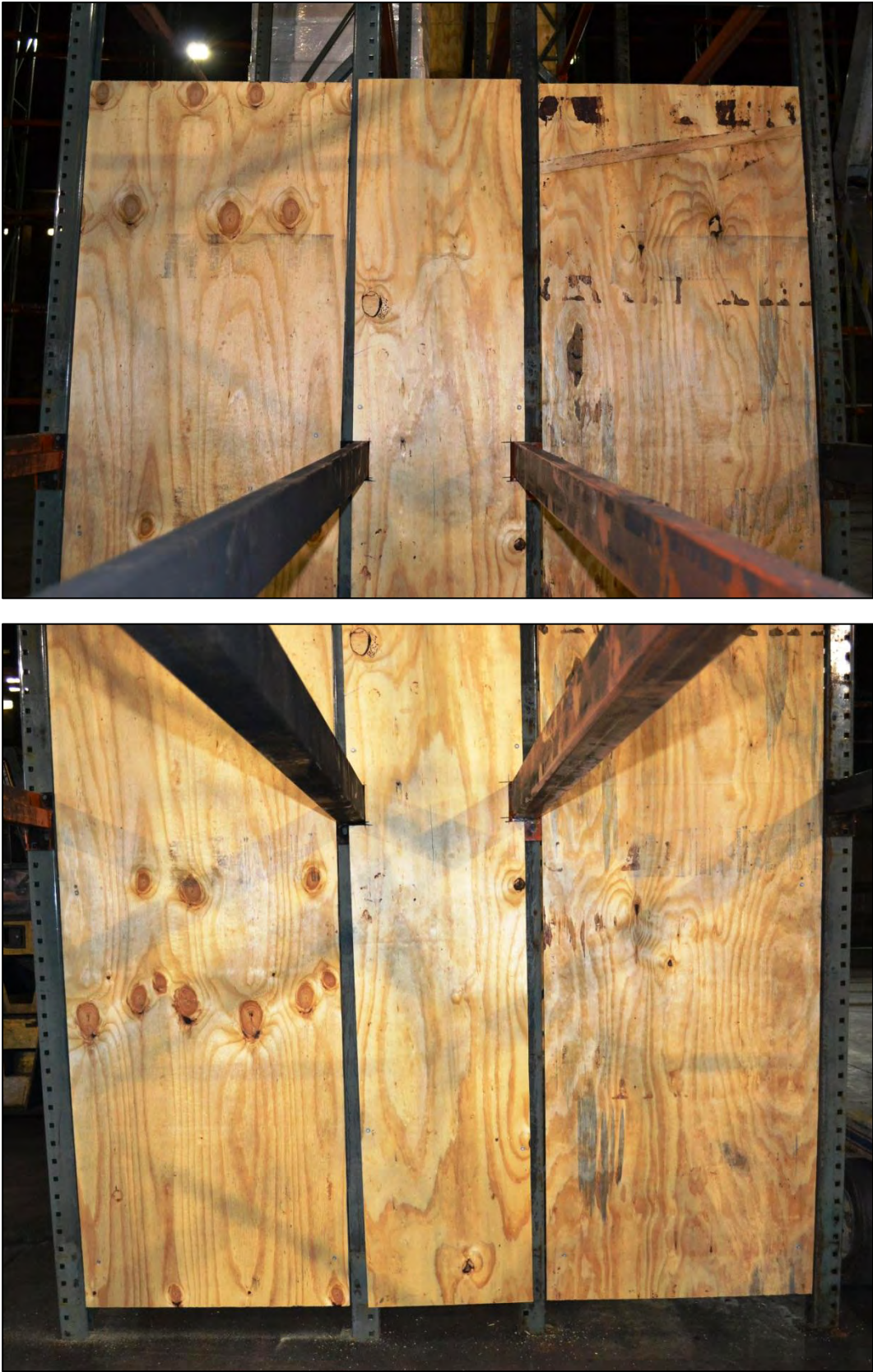
Figure 9 Combustible Vertical Barrier Detail
