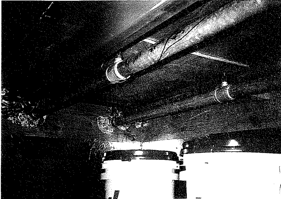
Photo 1 Sprinkler Test No. 1 Lower Tier Sprinkler Locations
