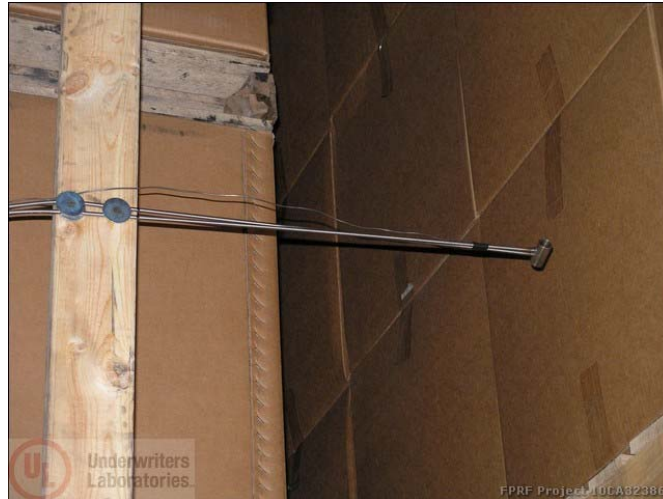
Figure 7 Representative Velocity Probe Installation
