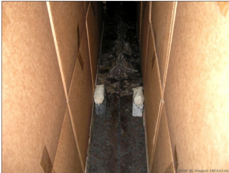
Figure 32 Test 5 Ignition Detail
