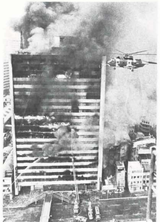
Fire initially spread through lower floors and the 21st floor. Middle floors were involved in the afternoon. Note streams from the 100-foot aerial and elevated platform.
