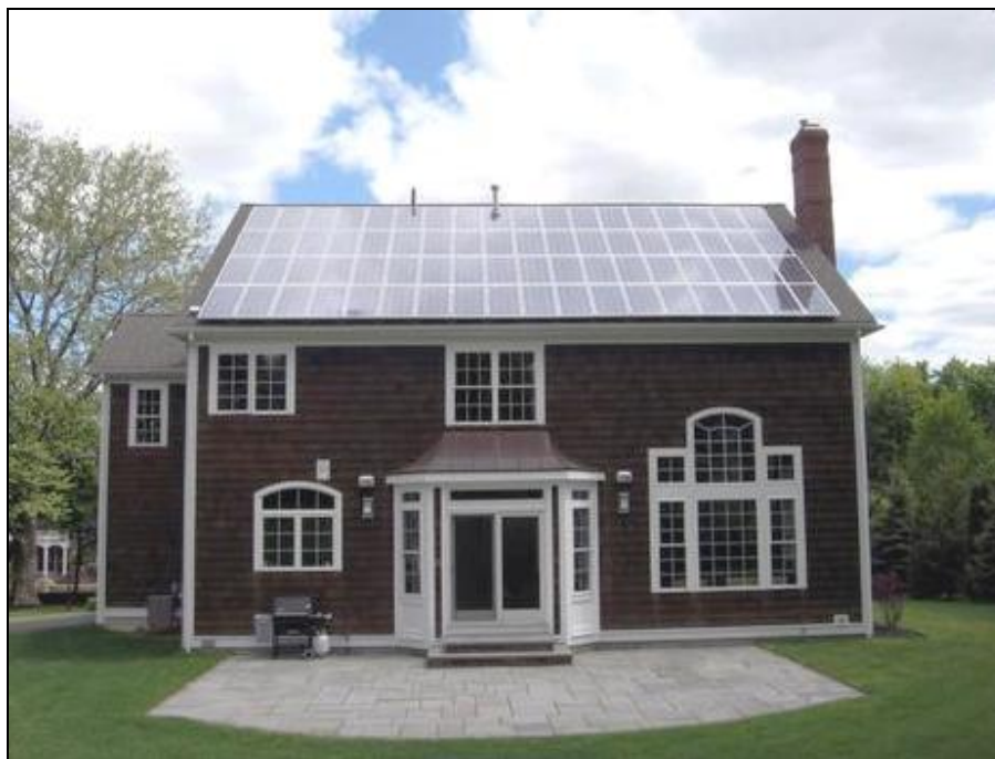
Figure 1-1: Example of Home with a Photovoltaic Solar Power System in Milton, MA (Photo courtesy of NREL Photographic Information Exchange)
