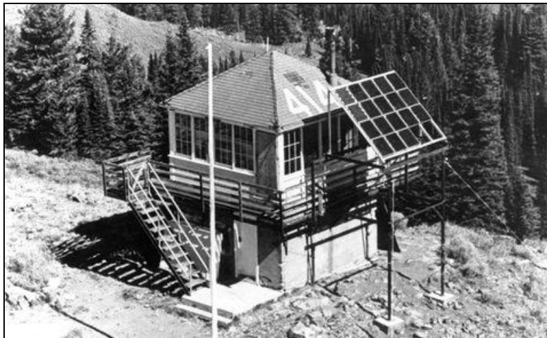
Figure 2-8: Example of PV System at a Remote Fire Lookout Tower in Idaho (Photo courtesy of NREL Photographic Information Exchange)
