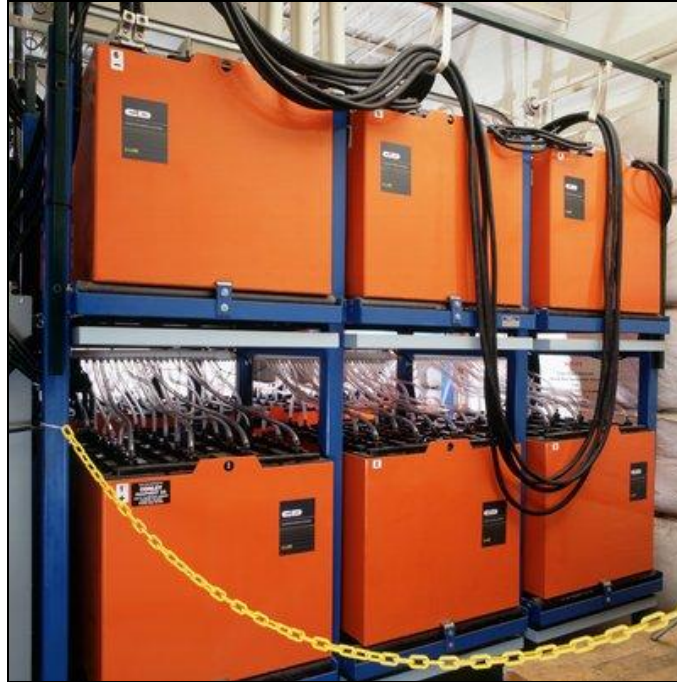
Figure 5-6: Typical Battery Installation for a Photovoltaic Solar Power System (Photo courtesy of NREL Photographic Information Exchange)
