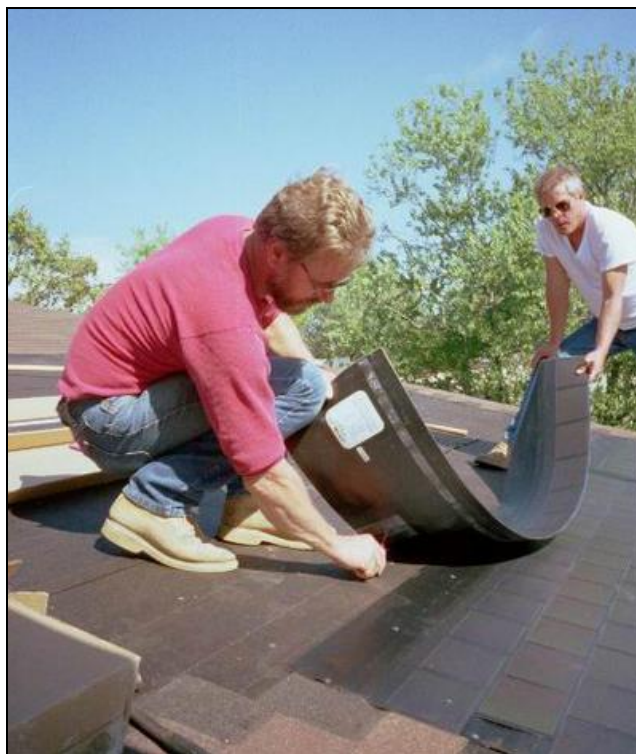
Figure 5-7: An Example of PV System Integral with Building Components (Photo courtesy of NREL Photographic Information Exchange)
