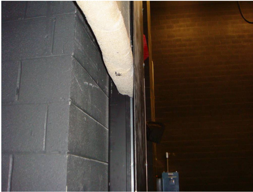
Figure C13 – Fire safety curtain during deployment
