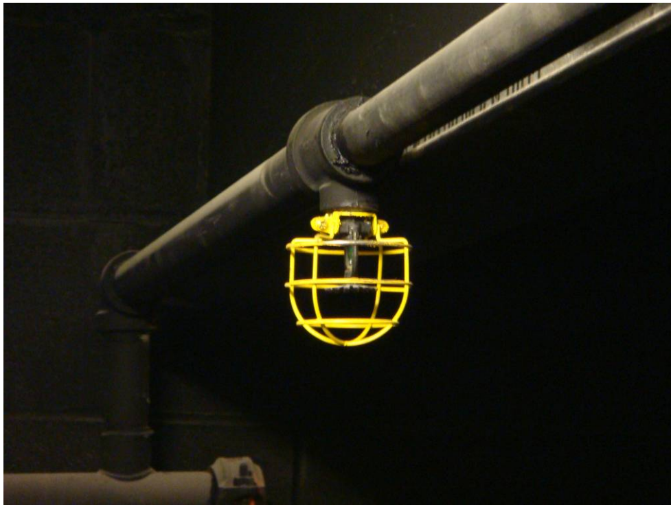
Figure C6- Sprinkler below ceiling(above gridiron)
