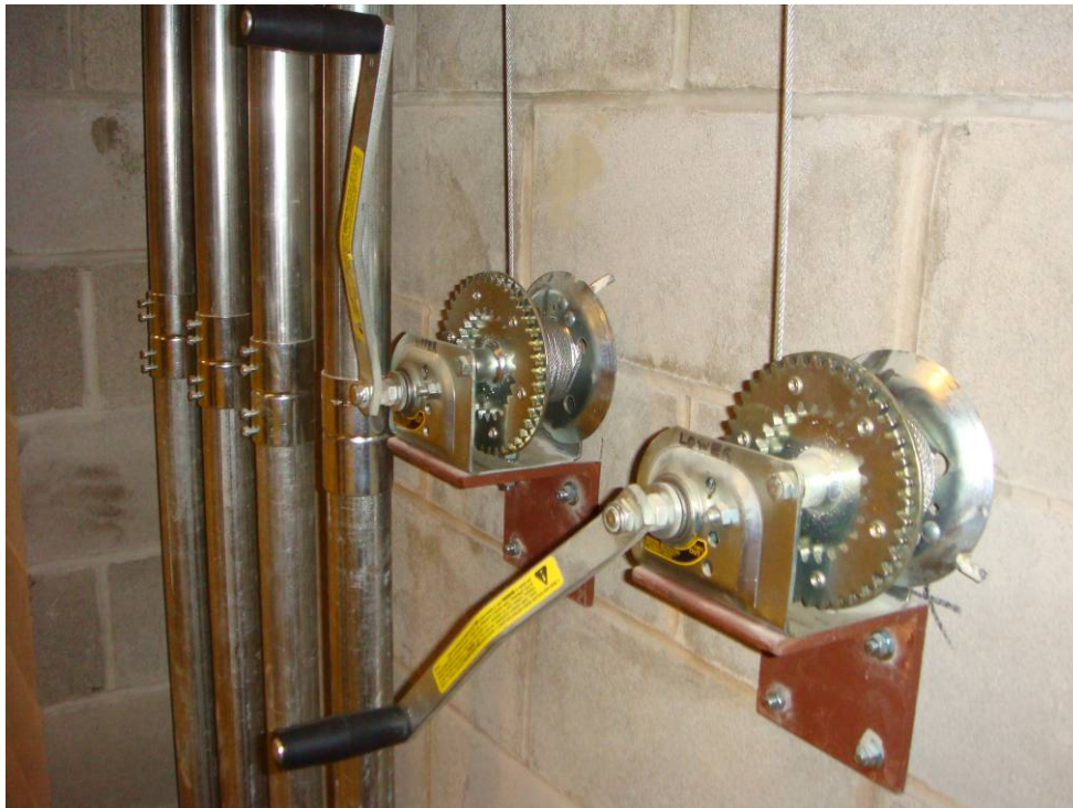
Figure C16– Manual control means for roof vent
