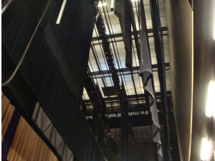
Figure C1- View up through flytower from stage
