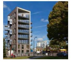
CLT construction was chosen over steel and concrete due to weight concerns as a storm relief sewer is located under the site. The use of CLT allowed the building to be lightweight, and prefabricated panelized construction resulted in a construction time of 10 weeks, less than half the estimated time for a concrete structure (Birch, 2011).
