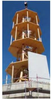
Completed in Hannover, Germany in 2012, TimberTower is a wind turbine constructed of glulam prefabricated panels that were assembled onsite (Quick, 2012).
