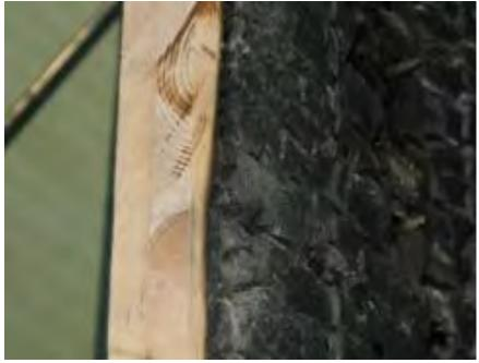
Despite the inherent fire resistance of heavy timber CLT panels, CLT elements are often required to be encapsulated by non-combustible gypsum board protection. This is intended to protect exposed CLT panels from heating and combustion and increase the fire resistance rating of the structural assembly. An example of gypsum board protection for a CLT wall is shown in the figure below.
