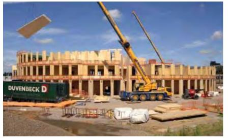
Figure 36 – Lifting prefabricated CLT panels for assembly (Crespell & Gagnon, 2010)
