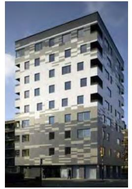
The prefabricated CLT panels allowed a team of four carpenters to construct the super-structure in less than four weeks (Waugh, Wells, & Lindegar, 2010).
