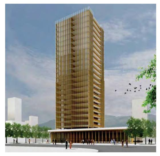
The structural system is based on a CLT core with steel beams supporting a timber floor slab. While the report highlights the need for fire engineering analysis, the report also presents fire performance solutions including charring and encapsulation approaches, in addition to fire alarm, detection and automatic sprinkler protection systems. To date, the Case for Tall Wood represents the most ambitious and comprehensive design for tall timber construction.
