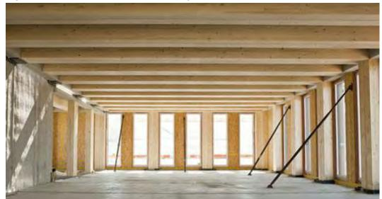
Figure 32 – Post and beam construction (Lignum, 2010)
