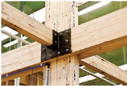
Figure 28 – Glulam beams and column (WoodSolutions, Glulam, 2013)
