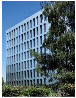
The Life Cycle Tower structural design is based on post and beam construction with large internal and perimeter glulam columns. These are combined with a concrete core for stability and hybrid timber-concrete floor slabs for fire separation and acoustic performance (Wurm, Gockel, & Unger, 2012).
