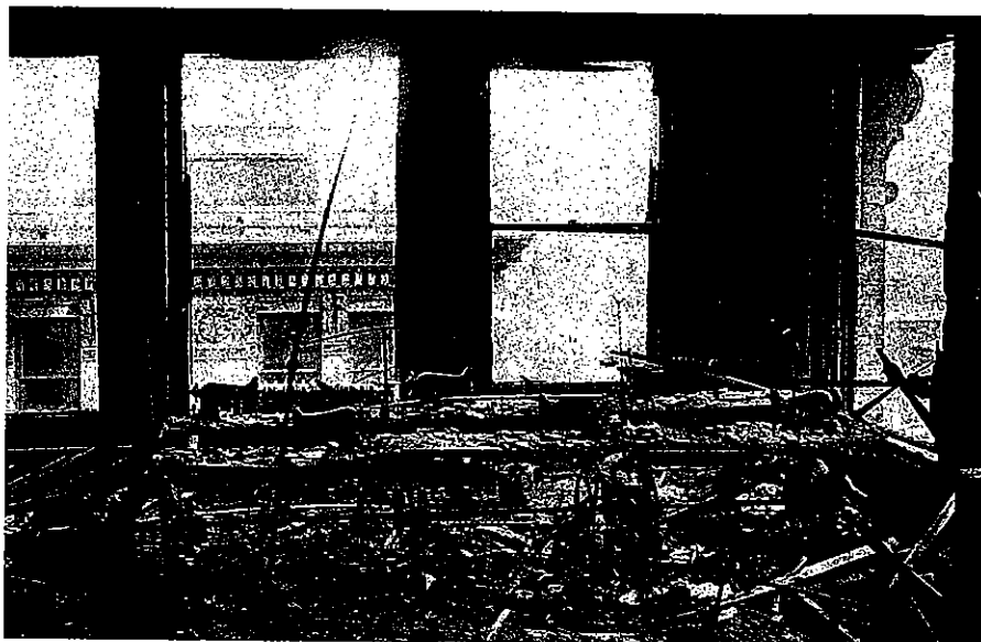
Within 30 minutes, the fire was under control. After 6:00 p.m., fire fighters began searching the top floors. They found incinerated victims on the ninth floor.
