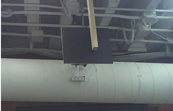
Figure 5. Photograph of the baffle and light source mounted in the ceiling.
