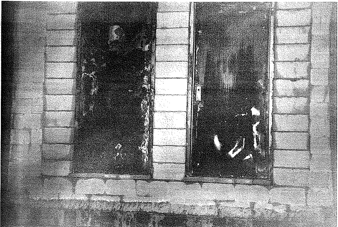
EXPOSED SIDE AFTER HOSE STREAM TEST
