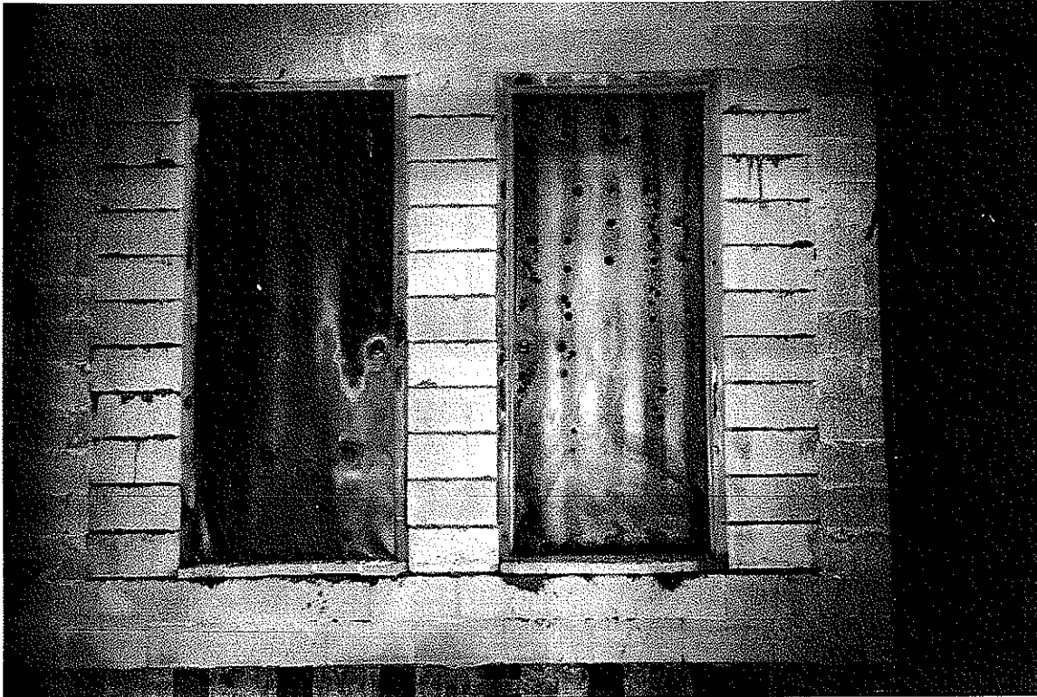
EXPOSED SIDE PRIOR TO HOSE STREAM TEST
