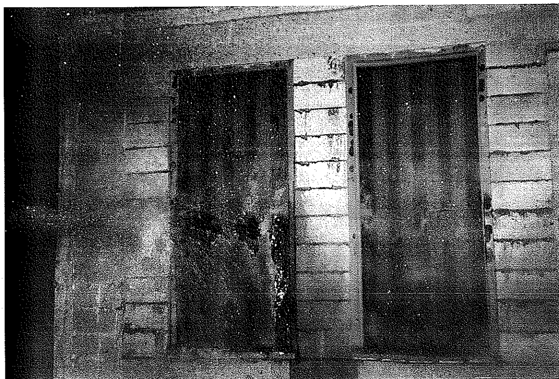
EXPOSED SIDE DURING HOSE STREAM TEST
