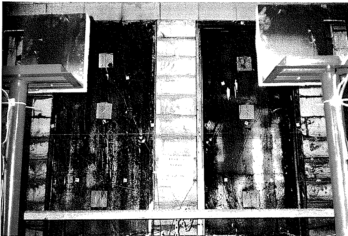
UNEXPOSED SIDE DURING FIRE TEST
