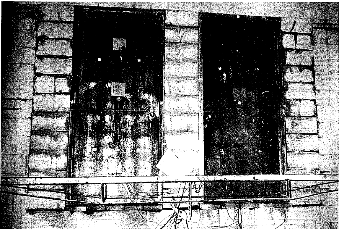
UNEXPOSED SIDE AFTER HOSE STREAM TEST
