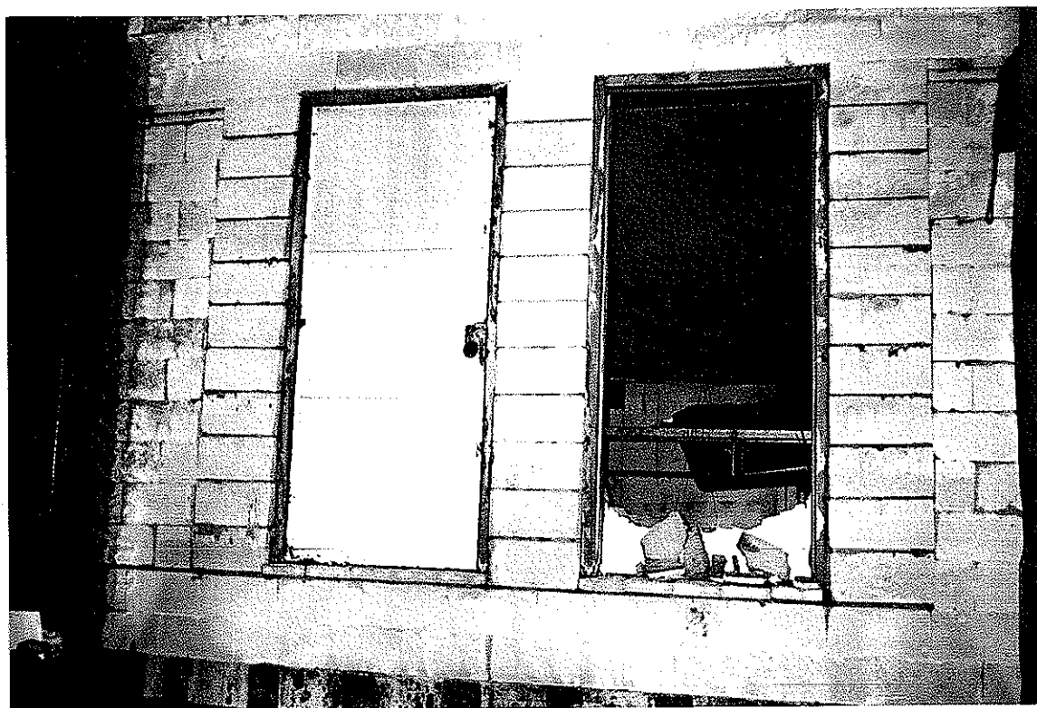
EXPOSED SIDE AFTER HOSE STREAM TEST
