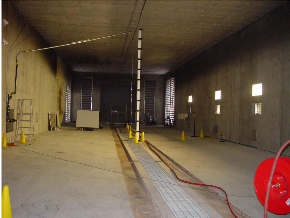
Figure 2.2. View of the East end of the tunnel facility
