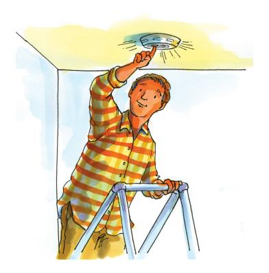
Wireless interconnection of smoke alarms is also available and can be installed by the homeowner.
