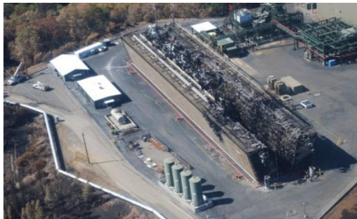
Figure 24 Aerial photo of destroyed cooling tower.
