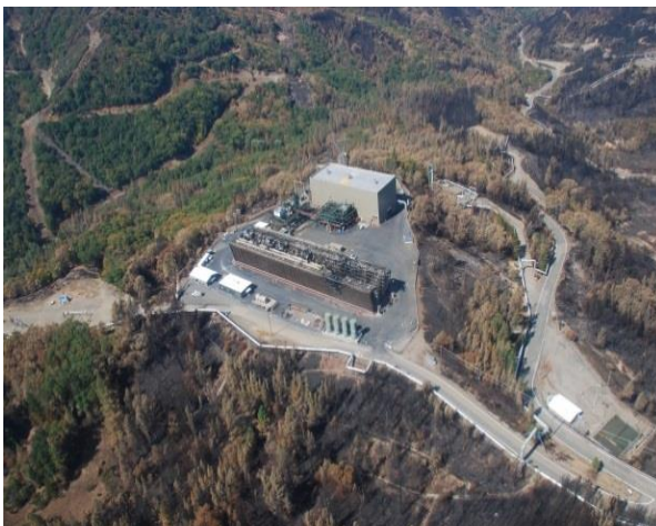
Figure 22 Aerial photo of destroyed cooling tower.
