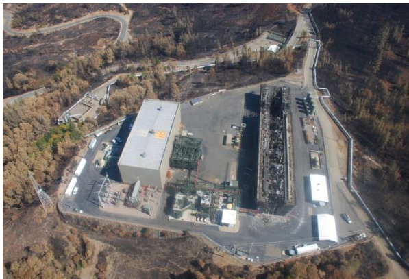
Photo 3: The Geysers power plant.
