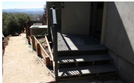
Photo 29 Non-combustible decking and clearance around and under the deck.
