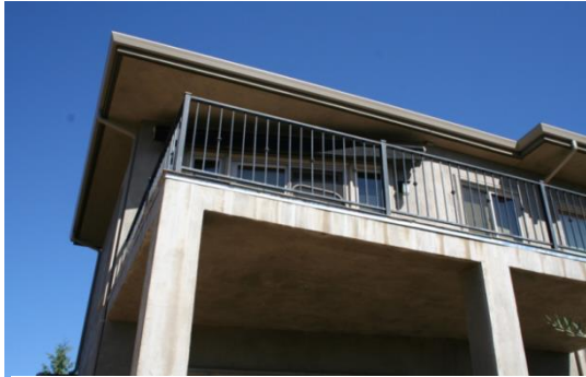
Figure 30 Non-combustible siding and windows.
