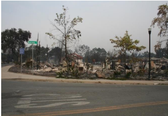
Figure 20 Middletown Manor apartment complex (after
