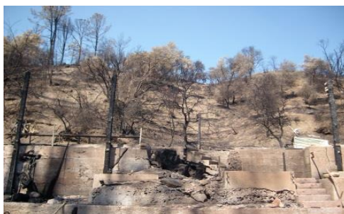
Figure 17 Multiple destroyed mid-slope structures.
