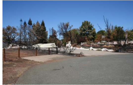
Figure 31 Street view of area structure damage.
