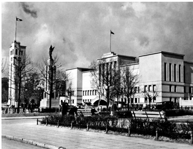
The Vytautas the Great War Museum opened in 1935. Architect Vladimiras Dubeneckis. Photograph by Vytautas Augustinas.
