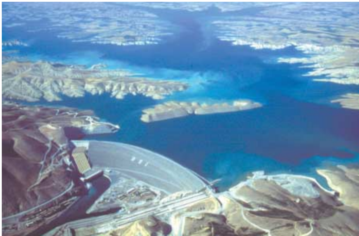
Fig. 1 - Keystone of the GAP project, the Ataturk dam has a reservoir capacity greater than Euphrates total annual flow which, as a result, has significantly transformed basin ecology.
