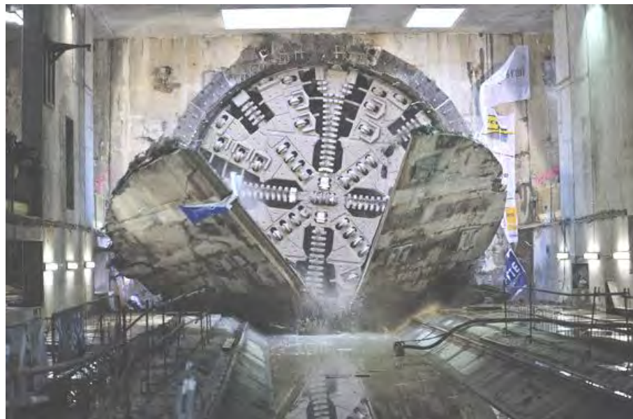
Figure 4-13. TBM arrival to the exit shaft
