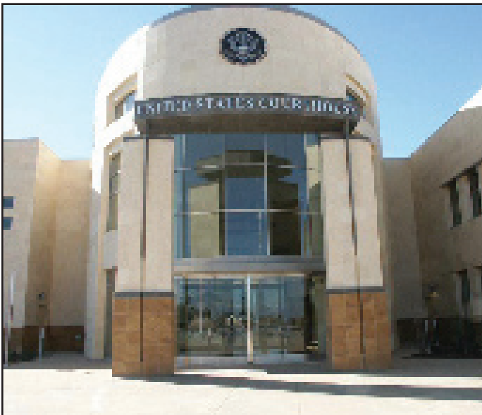
The U.S. courthouse in El Centro houses magistrate judges for the Southern District of California.
