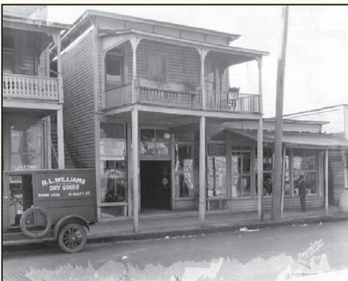
1111 East Scott Street, located on the south side of Scott Street just south of the new skate bowl (1927).
