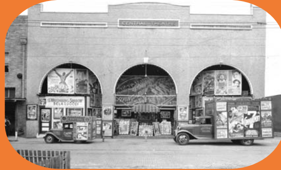
Central Theatre, 1201-03 Central Avenue, front facade with movie posters and advertising trucks, 1934 Photo from Tampa Bay History Center
