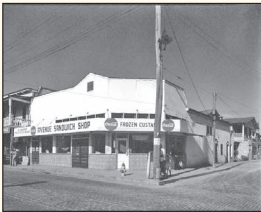
Central Avenue Sandwich Shop, 1301 Central Avenue, east side of Central at the former intersection with Constant Street, now approximately Laurel Street/Ray Charles Boulevard (1949).
