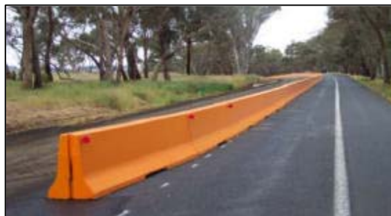
Examples of safety barriers (from VicRoads' Road Design Note 912A), above (Current at October 2005 version of Road Design Note.)
