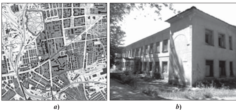
Fig. 3. Workers' industrial settlement "Carbide Colony" situated near the carbide factory: a) general layout of the settlement; b) a former kindergarten on the Pantchenko St.
