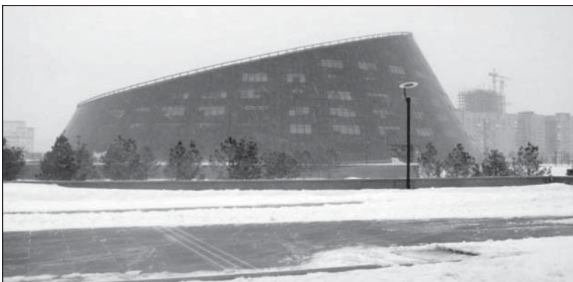
Photo 1. Perspective view of side face of “Shabyt” Palace of Arts, 2009
