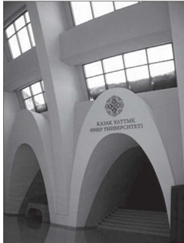
Photo 14. Corbel arched doorways – entries to the audience hall
