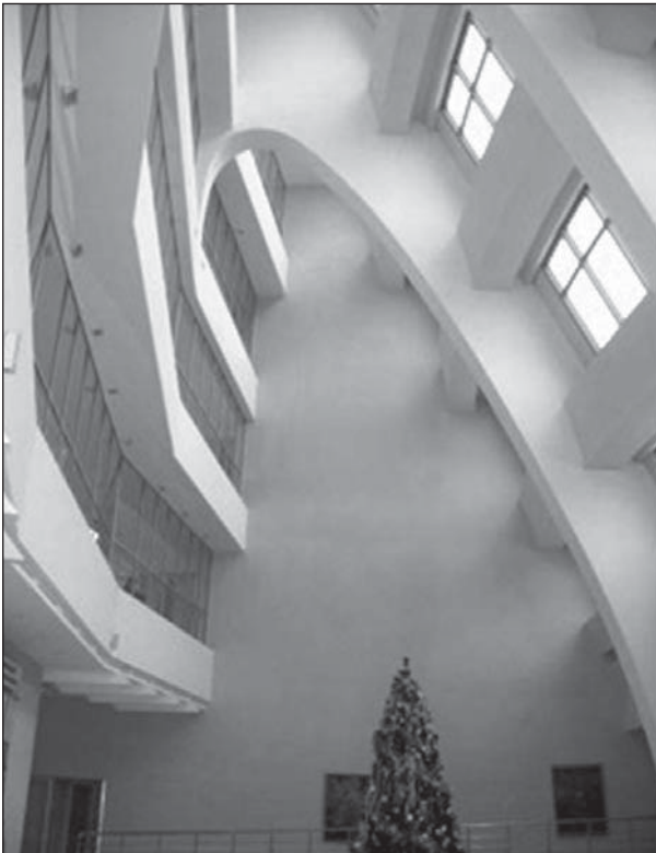
Photo 13. Interior of corbel lancet arches in the lobby opposite the assembly hall
