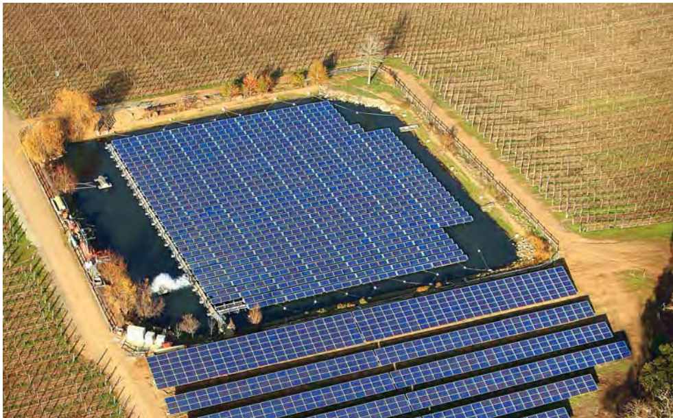
200kW Installation at Far Niente
