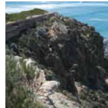
Cliff erosion at Barwon Heads Photo: Catharina Greve
