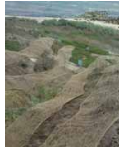
Jute matting erosion control, Curlewis, Corio Bay Photo: Matt Crawley, Bellarine Catchment Network
