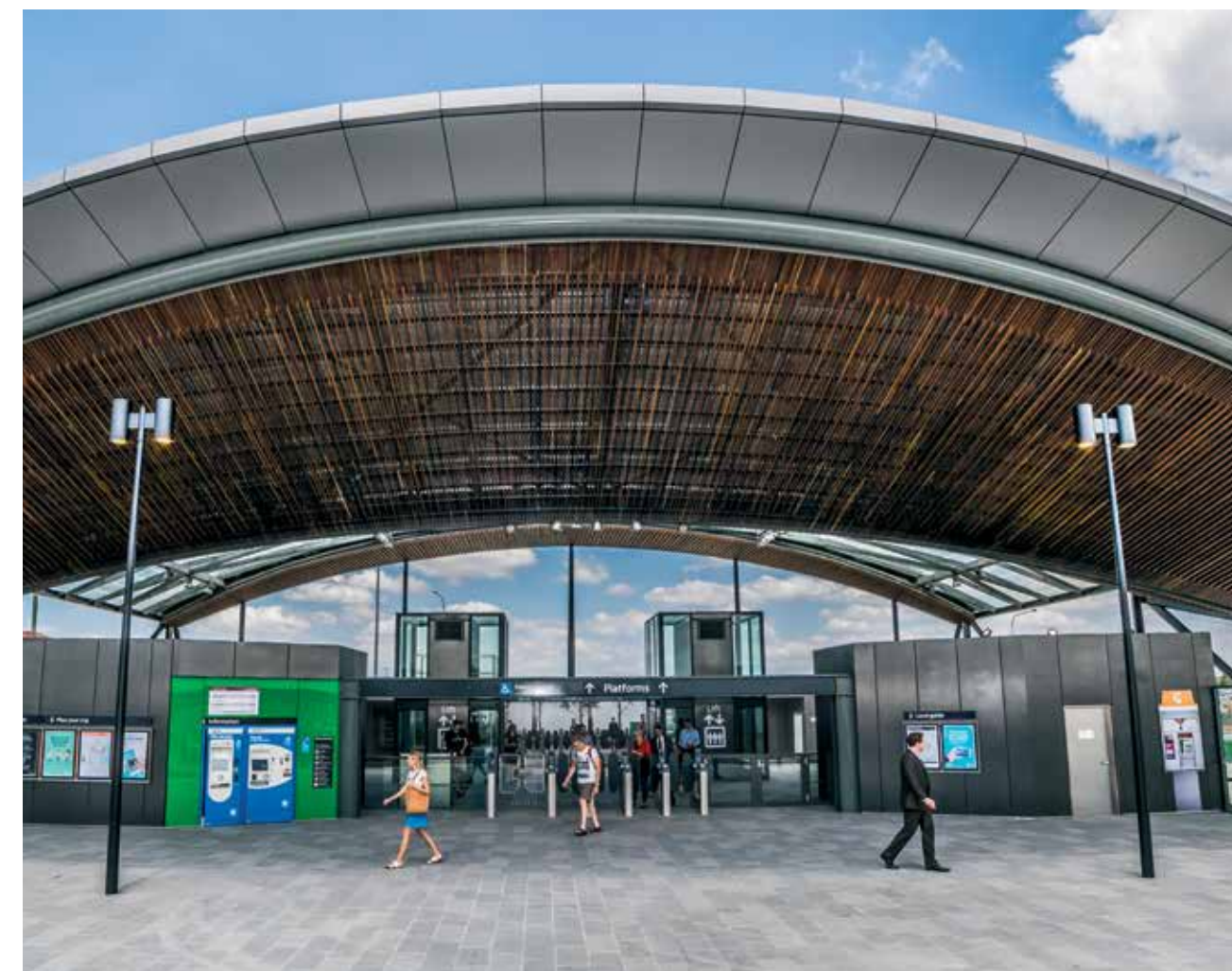
Sydney Metro Northwest prototype station
