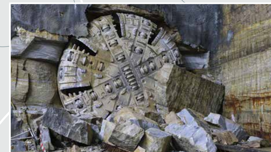
TBM2 Florence break-through at Showground, June 2015
