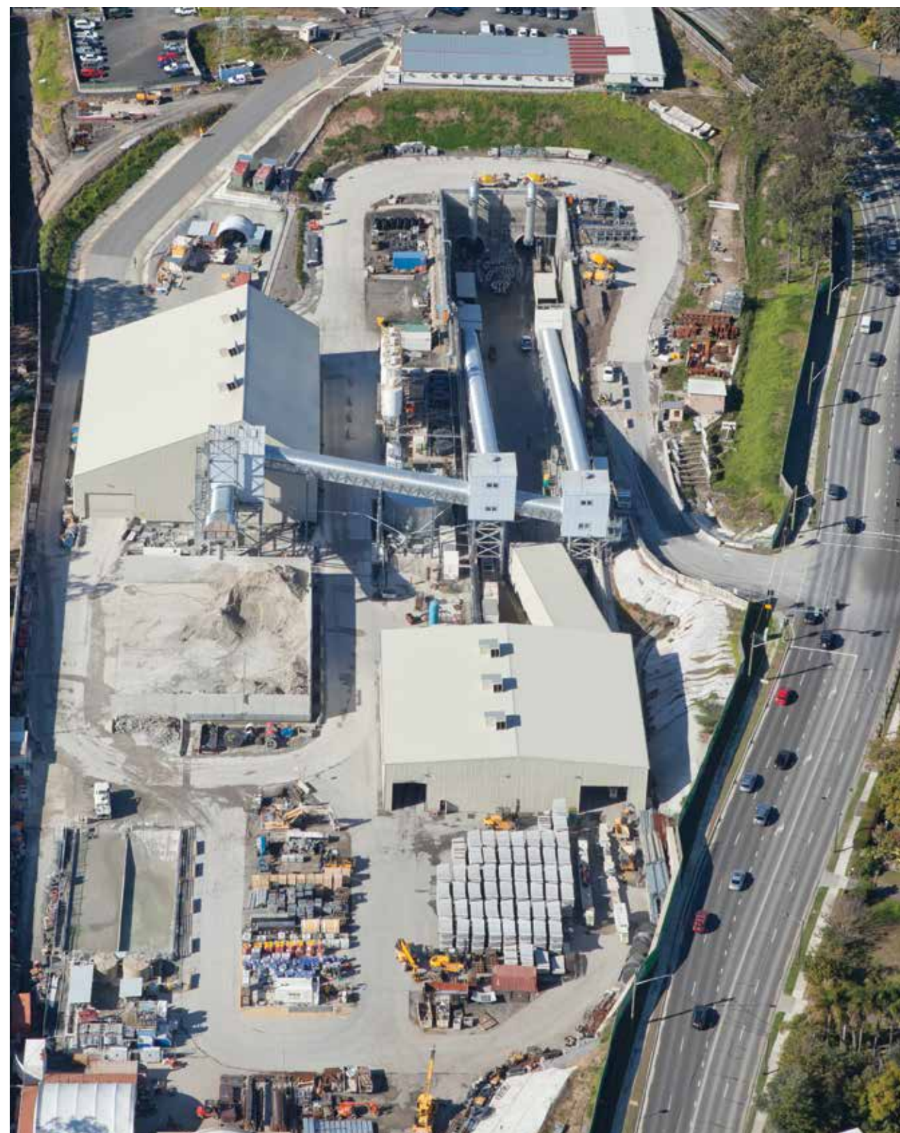
Cherrybrook Station TBM dive site and tunnel portal, July 2015
