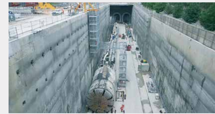
Following the first break-through, TBM Elizabeth traverses the Norwest Station site, February 2015
