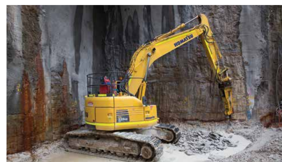
Excavator with rock hammer at the Epping construction site, April 2015
