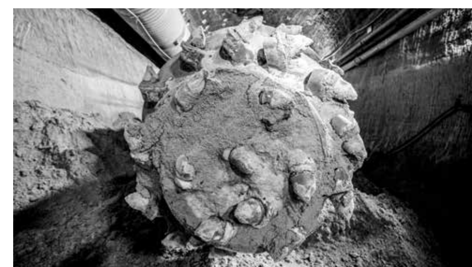
Roadheader excavating the crossover cavern at Epping, March 2015
