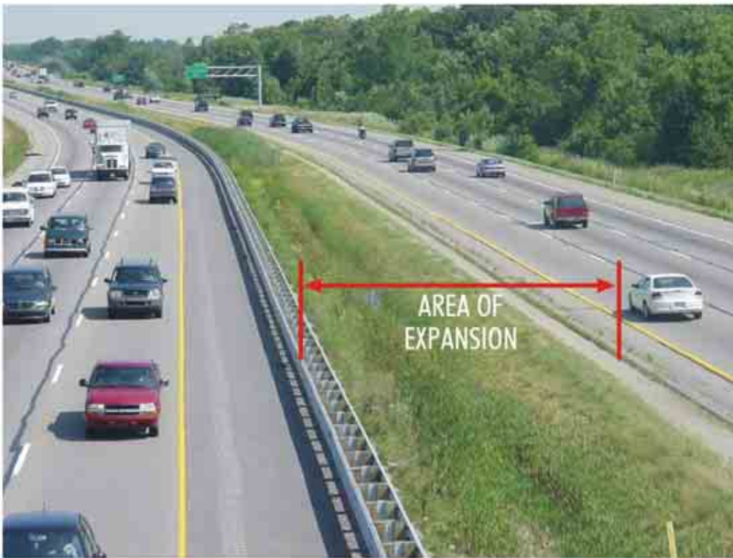
I-75 in At-Grade Freeway Section
