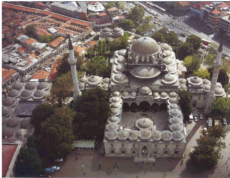
Figure 6 - General view of Bayzid II Mosque showing the prayer hall joined with the courtyard. The structures at the wings are the tabhane serving as accommodation for travellers. The minarets are unusually planted away from the mosque structure.
