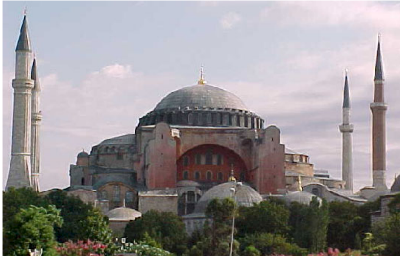
Figure 8 - Hagia Sophia (Istanbul, 532-37) exterior showing the structural composition and support of the dome.
