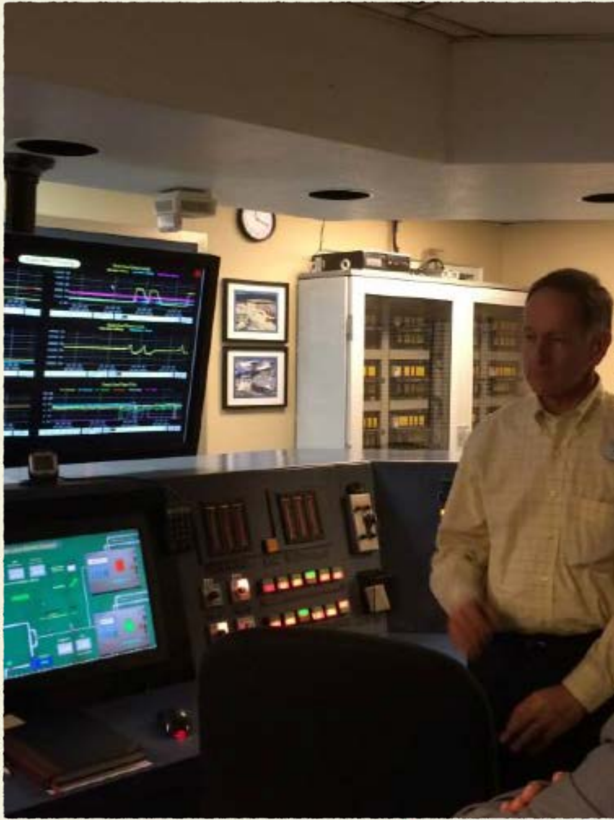
Water quality and systems for all Walt Disney World can be controlled from this room.
