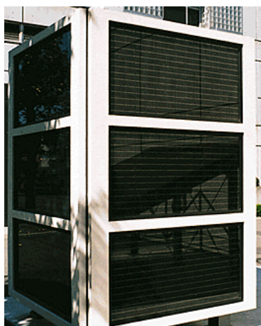
Figure 3.7 - Curtain walling detail
