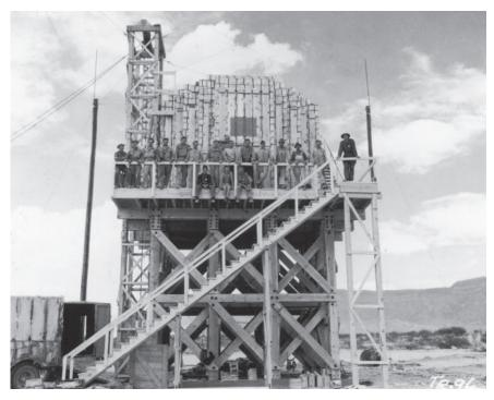
Workers on the Manahattan Project in Alamagordo shown on a platform stacked with TNT interlaced with fission products. Explosion of the TNT was meant to make sure measuring and observation equipment functioned and was correctly calibrated before the first test. Such testing also provided experience and built tacit knowledge in capturing data from an atomic test. Photo © Time&Life Pictures/Getty Images.
