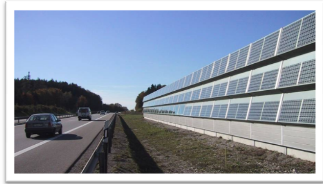
Figure 7-1: Soundwall in Germany
