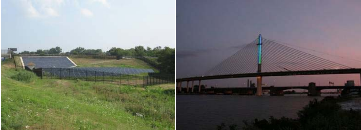
Figure 7-12: Veteran's Glass City Skyway 100-kW Solar Array and Lighted Pylon Source: Ohio DOT's Office of Public Communications
