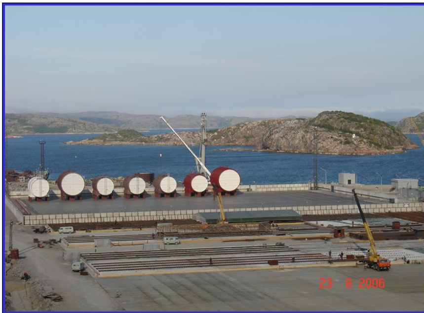
Figure 6. First bunch of reactor compartments delivered to Sayda Bay
