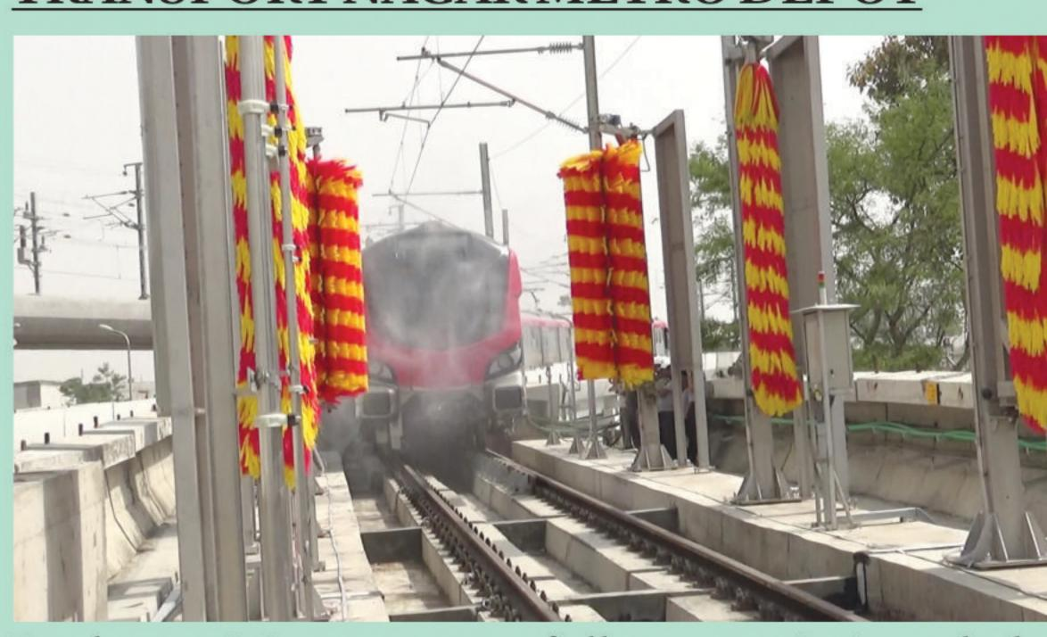
Lucknow Metro successfully commissioned the Automatic Train Washing Plant at the Transport Nagar Metro Depot on 28th April, 2017. Through this facility, the Metro trains entering or exiting the Depot can be cleaned automatically at the ramp using remote control from the Operation Control Centre (OCC) located inside the Depot.
