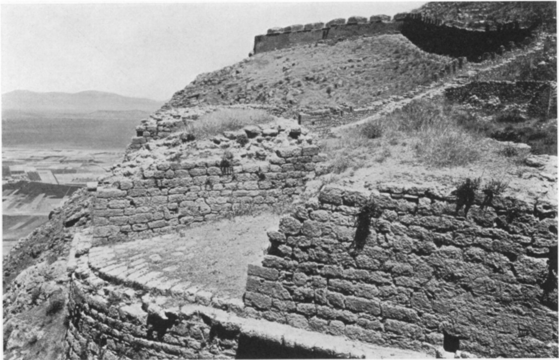
FIGURE 142. PLATFORM BEHIND NORTHWEST BASTION, THIRD LINE
