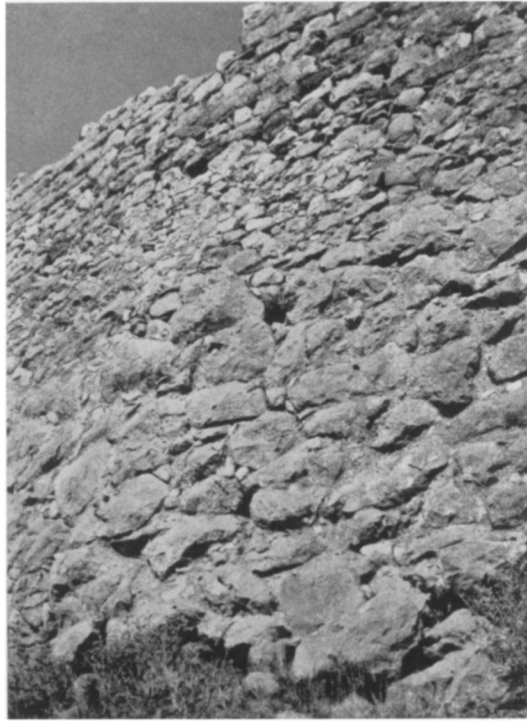
FIGURE 32. SOUTH CIRCUIT WALL: DETAIL FROM SECTOR 43-44
