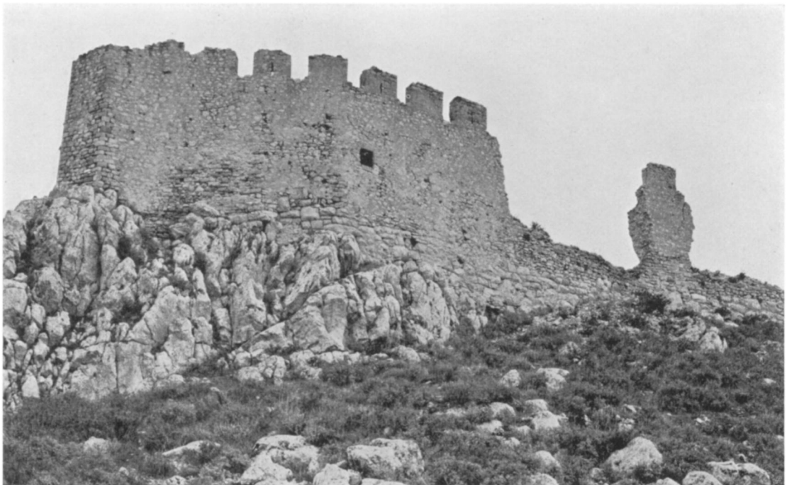
FIGURE 167. SAME, FROM WITHOUT, SHOWING NORTHEAST BASTION
