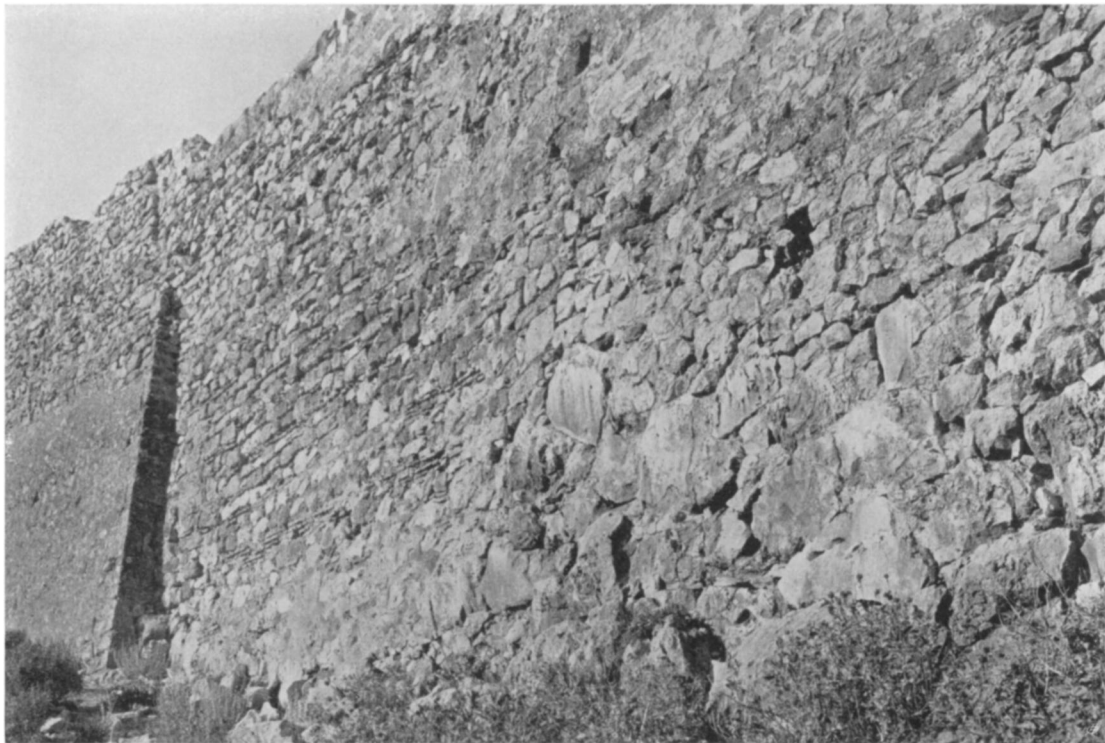
FIGURE 186. EXTERIOR FACE OF WALL, BETWEEN 40 AND 41
