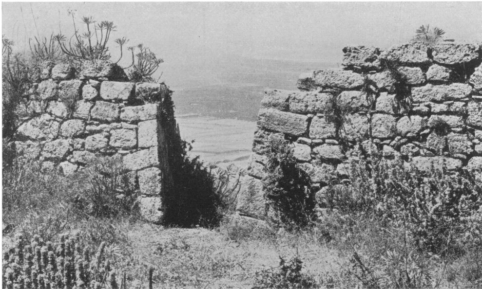
FIGURE 123. CANNON EMBRASURE, SOUTH LATERAL WALL OF THIRD LINE
