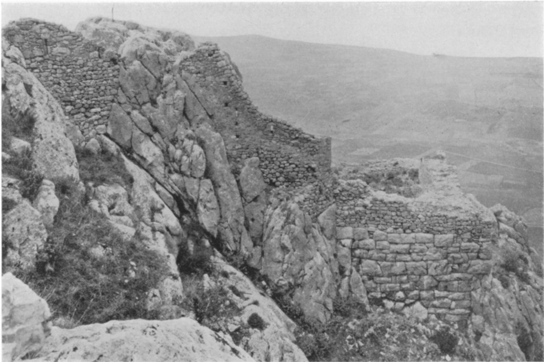
FIGURE 17. NORTH CIRCUIT WALL AT 17
