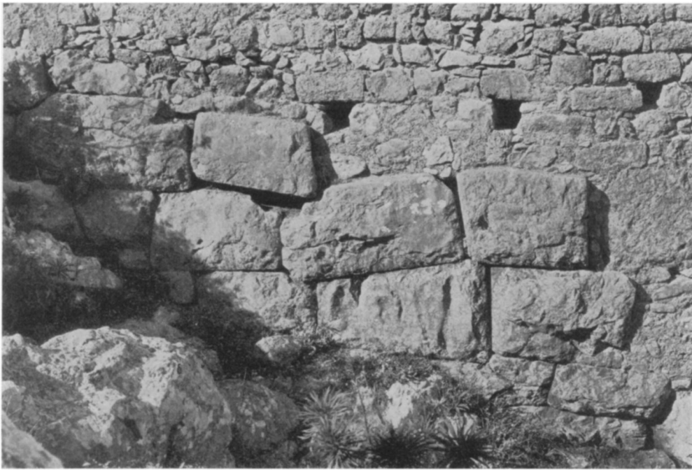
FIGURE 24. NORTH CIRCUIT WALL: INTERIOR AT 27
