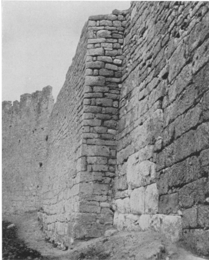
FIGURE 19. NORTH CIRCUIT WALL AT 20
