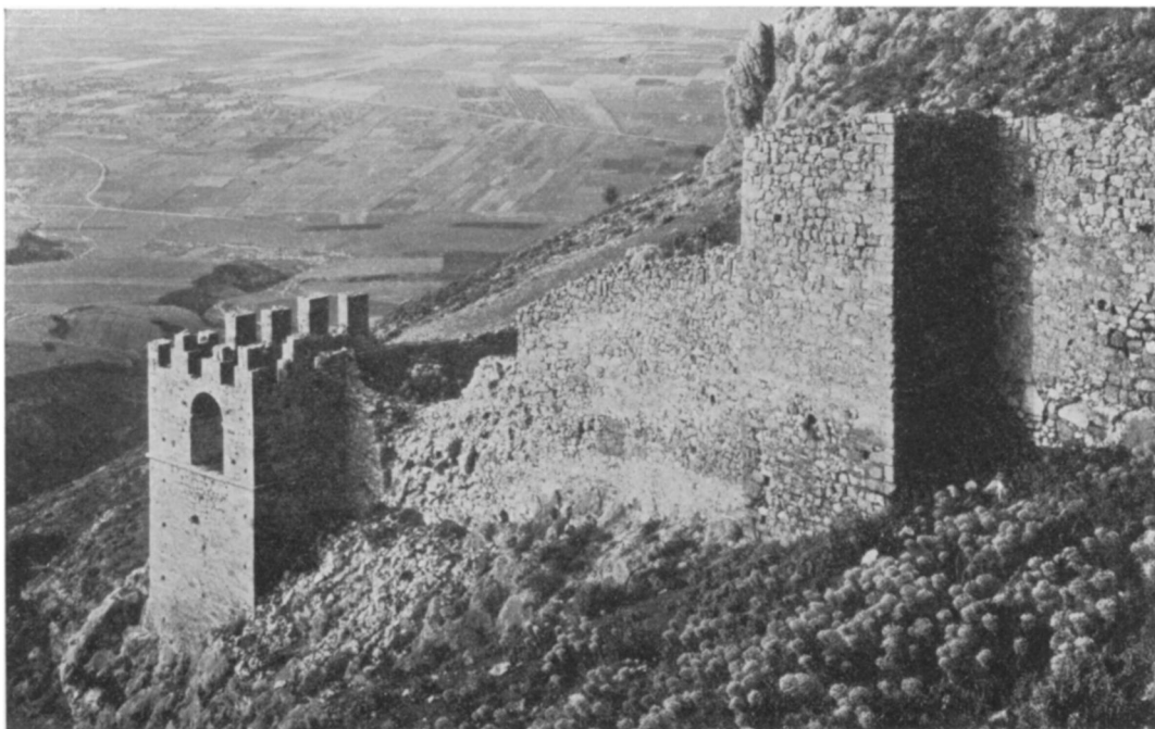
FIGURE 107. NORTH BASTION AND HOLLOW TOWER, FIRST LINE
