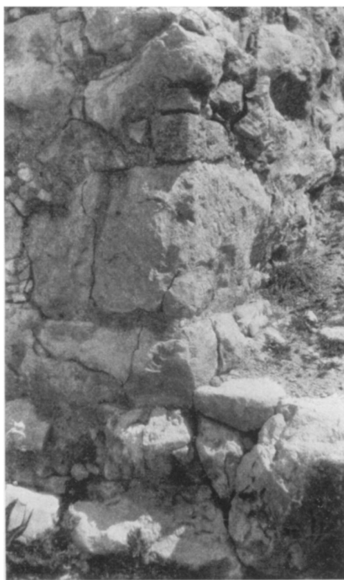
FIGURE 12. WEST DEFENSES: THE NORTH BASTION. JUNCTION WITH SPUR WALL
