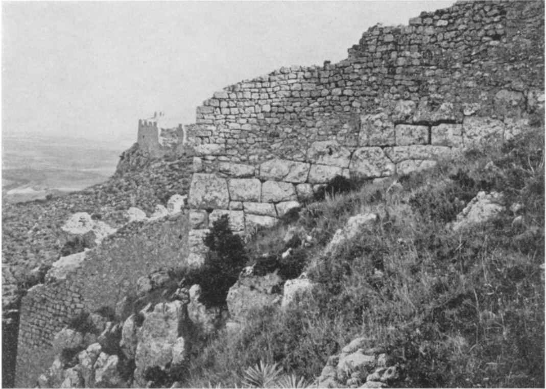
FIGURE 23. NORTH CIRCUIT WALL: EXTERIOR AT 27
