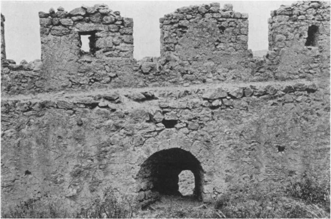
FIGURE 163. INTERIOR FACE OF WALL, BETWEEN 27 AND 28
