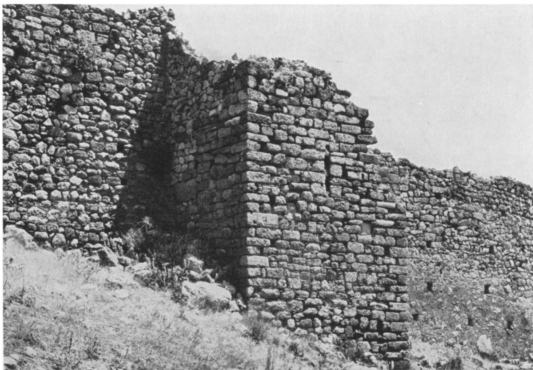
FIGURE 188. TOWER IN SOUTH WALL, AT 41
