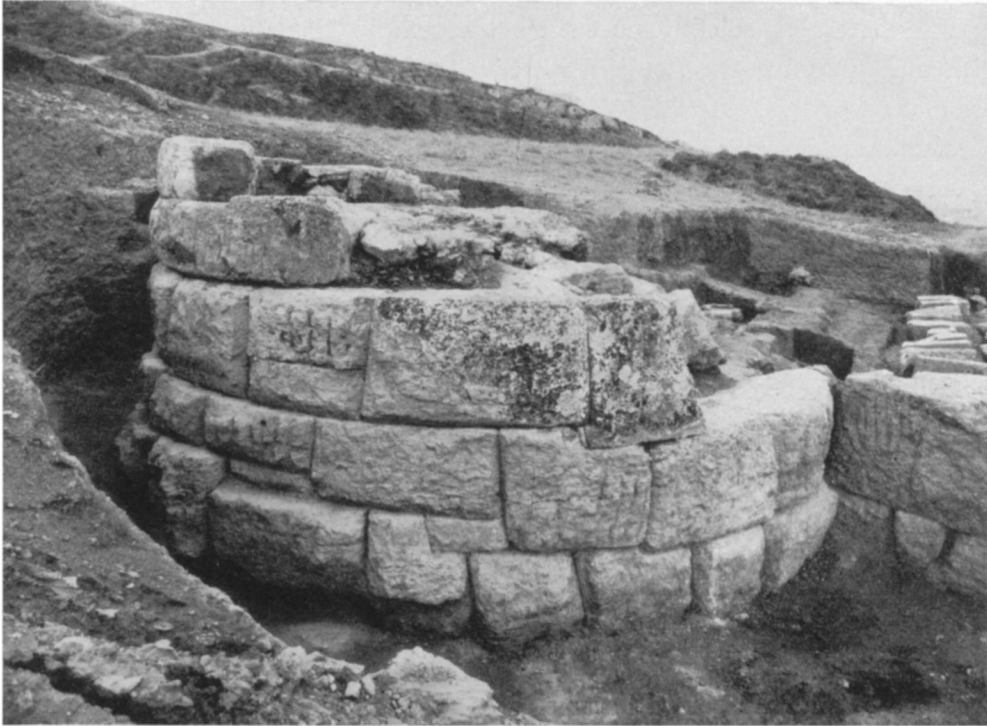
FIGURE 64. ISTHMIAN GATE: TOWER I FROM NORTHEAST
