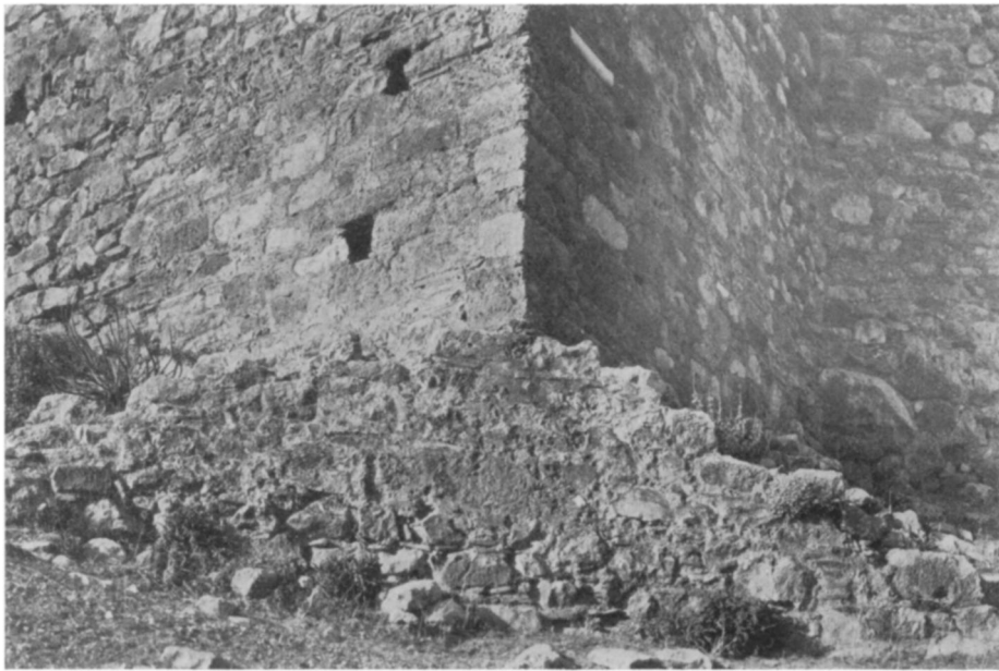
FIGURE 185. BASE OF TRIANGULAR BUTTRESS AT 40
