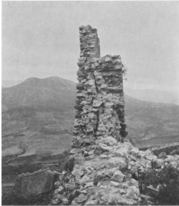
FIGURE 178. BREACH IN WALL, BETWEEN 33 AND 34
