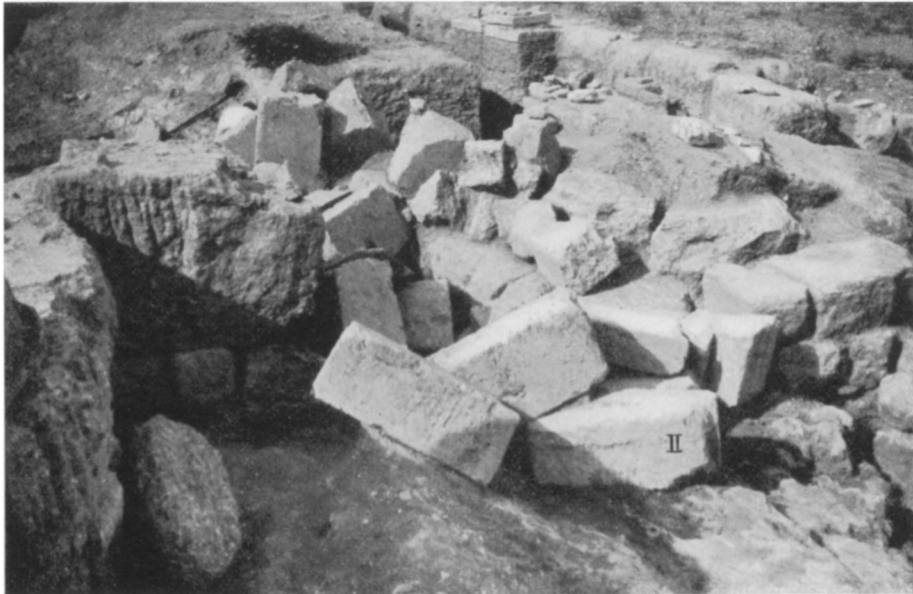
FIGURE 76. ISTHMIAN GATE: FALLEN VOUSOIRS IN OUTER ENTRANCE
