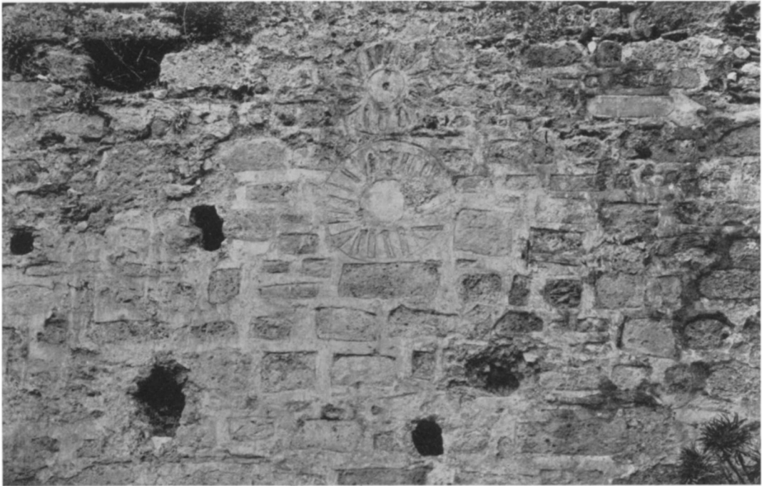
FIGURE 135. DECORATIVE REPAIRS TO THIRD LINE WALL
