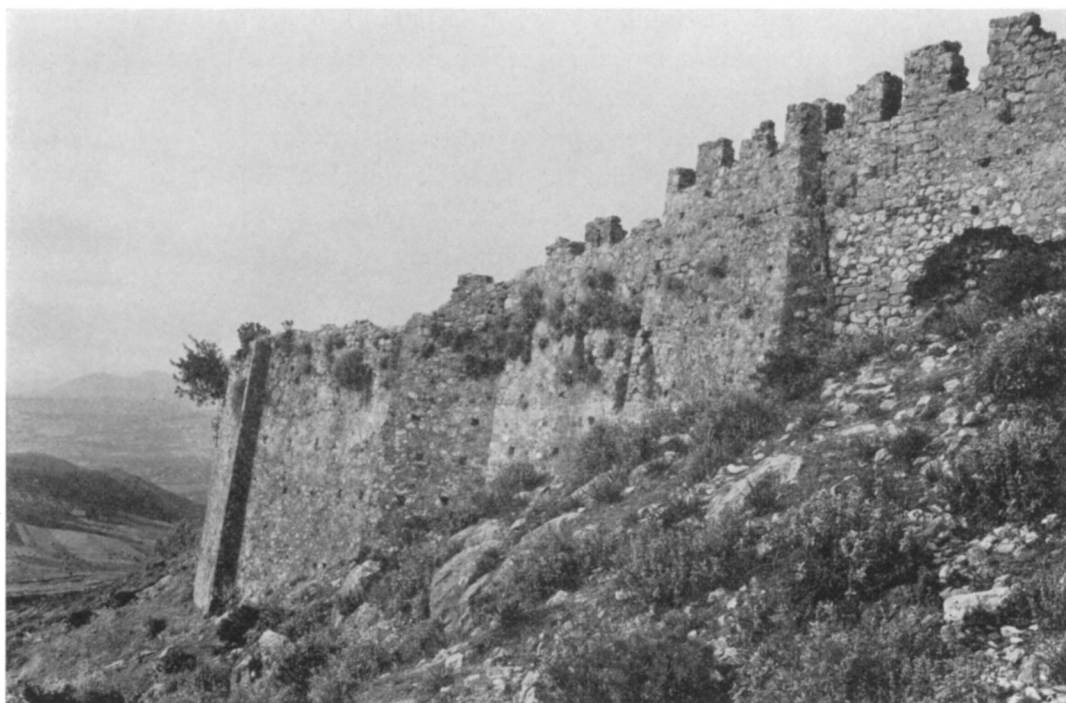
FIGURE 183. EXTERIOR FACE OF WALL, OPPOSITE PEIRENE
