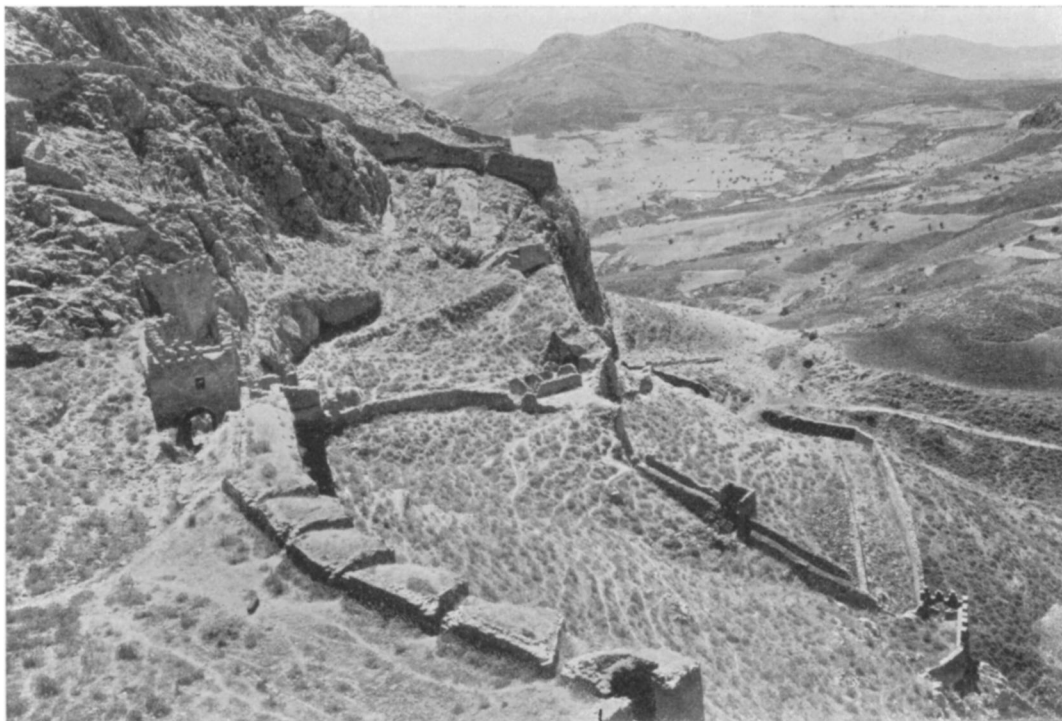
FIGURE 106. FIRST AND SECOND LINES OF DEFENCE, SEEN FROM WITHIN
