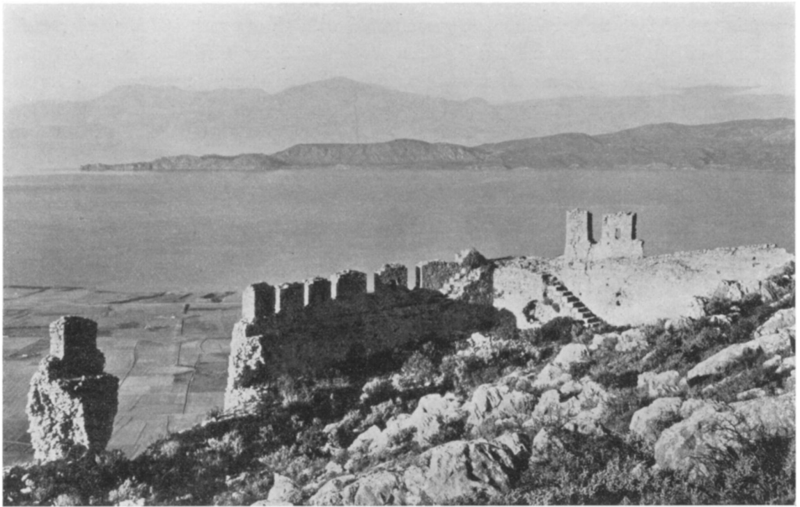
FIGURE 166. NORTHEAST ANGLE OF CIRCUIT WALL, FROM WITHIN (Through the breach, Venetian earthworks in the plain)
