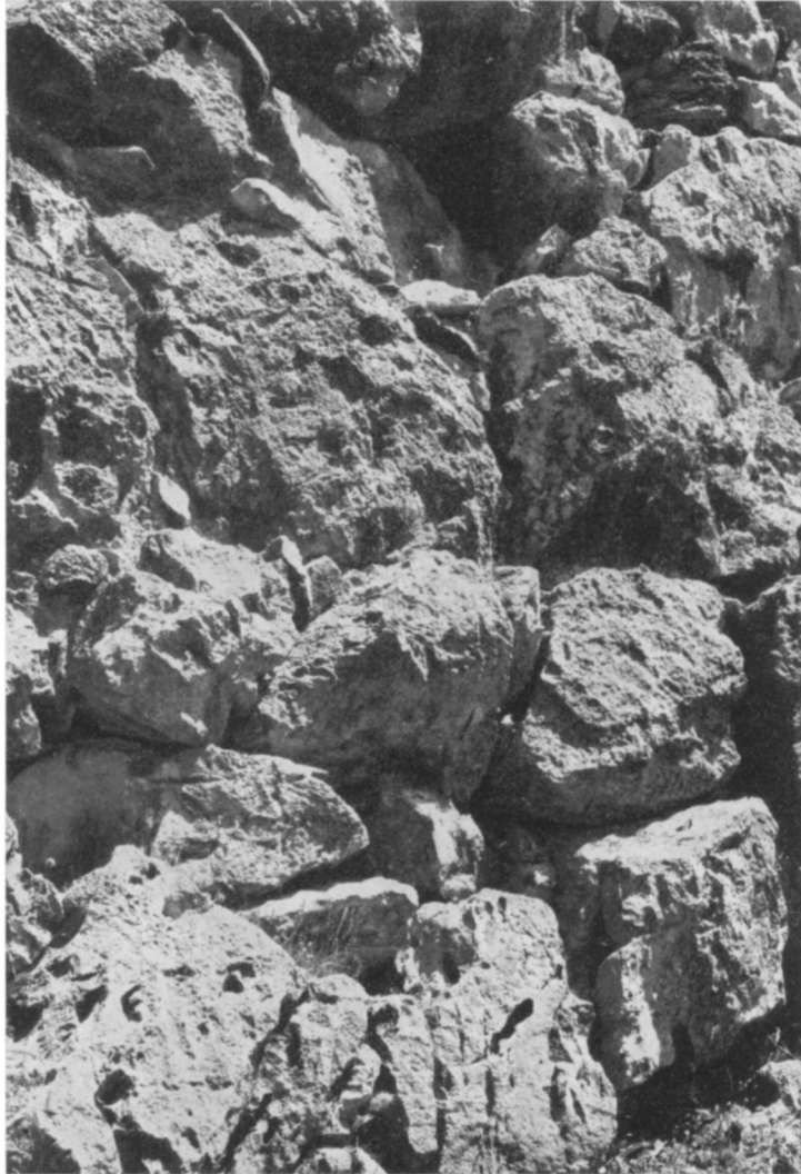
FIGURE 25. EAST CIRCUIT WALL: DETAIL OF CYCLOPEAN MASONRY
