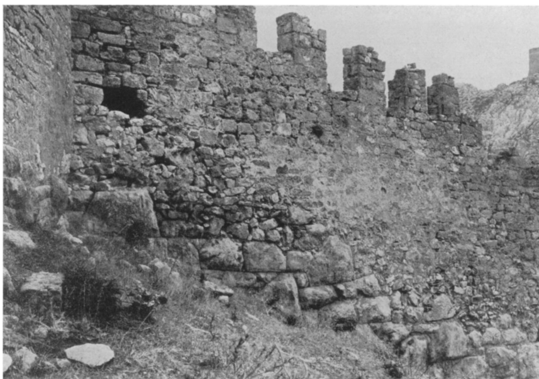
FIGURE 16. NORTH CIRCUIT WALL AT 14
