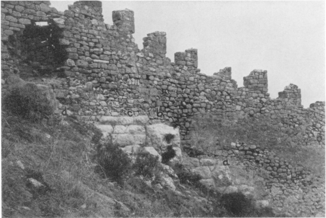
FIGURE 15. NORTH CIRCUIT WALL AT 13
