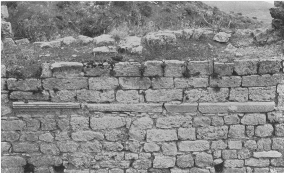
FIGURE 102. SOUTH WALL OF MOAT, SHOWING BRIDGE SUPPORT
