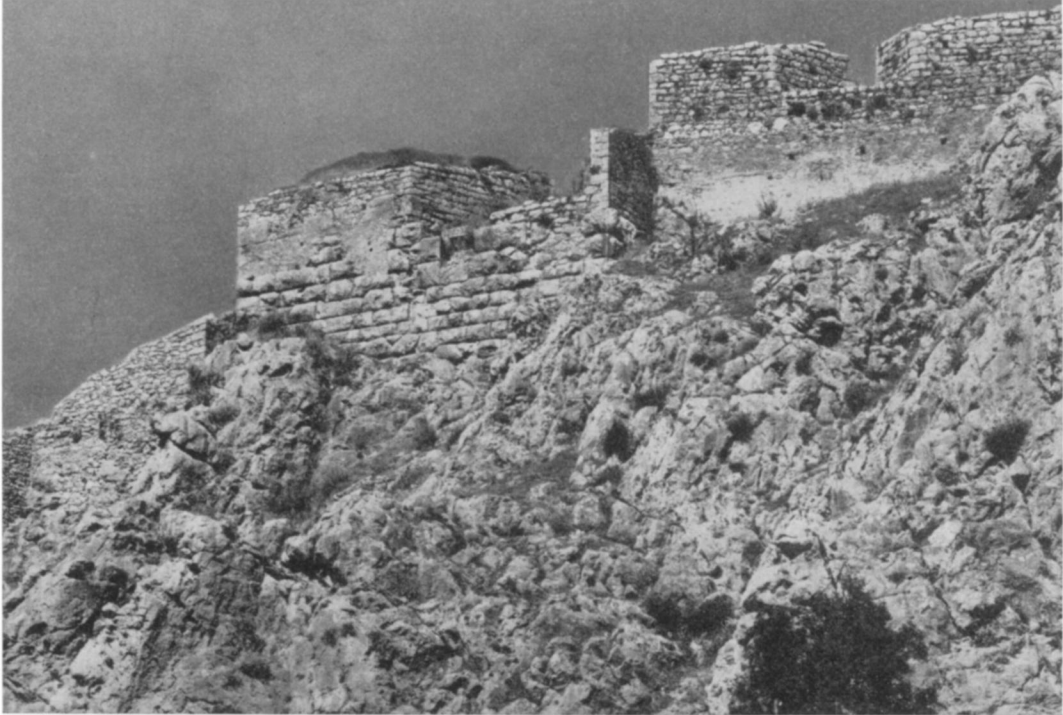
FIGURE 5. WEST DEFENSES: THE SOUTH BASTION, FROM THE WEST
