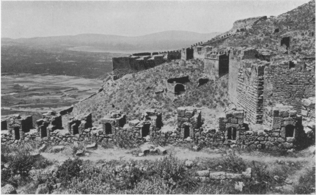
FIGURE 124. PARAPET AT EAST END OF SOUTH LATERAL WALL, THIRD LINE
