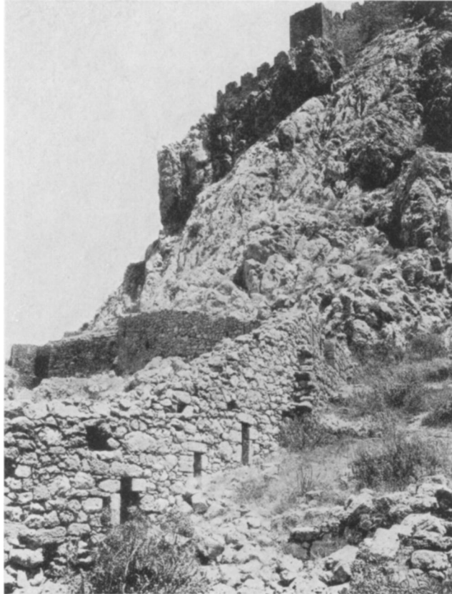
FIGURE 118. THIRD LINE: WEST EXTENSION, NEAR 4
