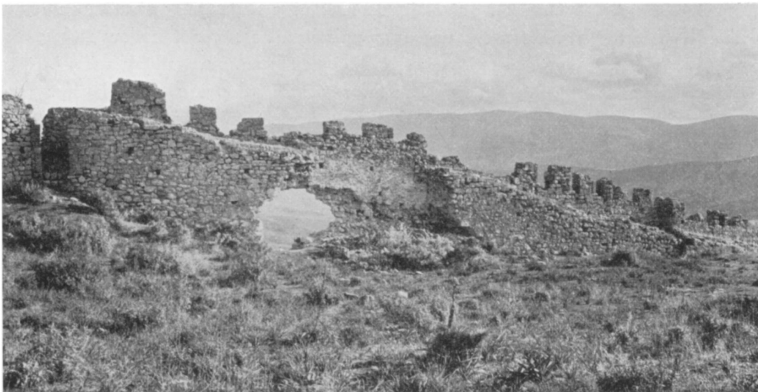
FIGURE 182. INTERIOR FACE OF WALL, 37-39, SHOWING TOWER AT 37
