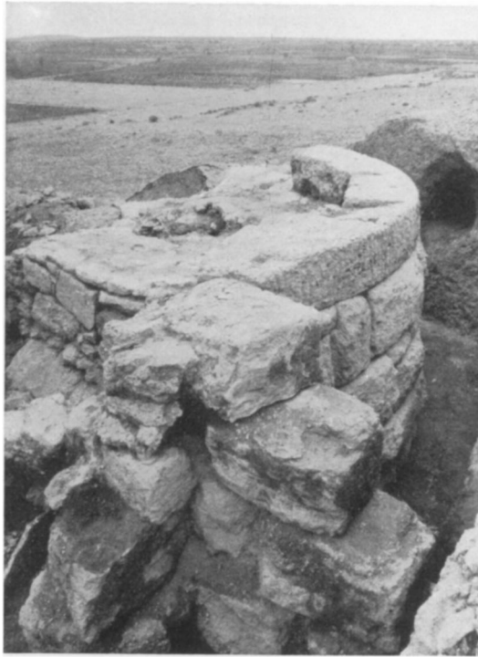
FIGURE 66. ISTHMIAN GATE: TOWER I FROM SOUTHWEST
