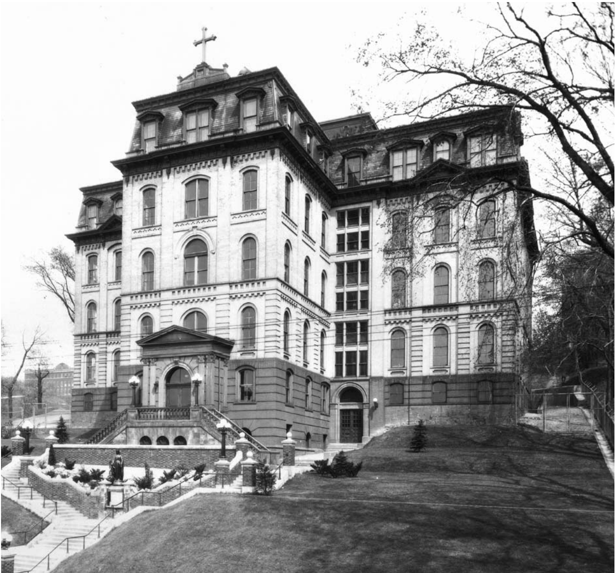
This 1932 photograph of the Catholic Central High School's west elevation illustrates the boys' entrance and southwest stairway addition. Courtesy of the Rensselaer County Historical Society.
