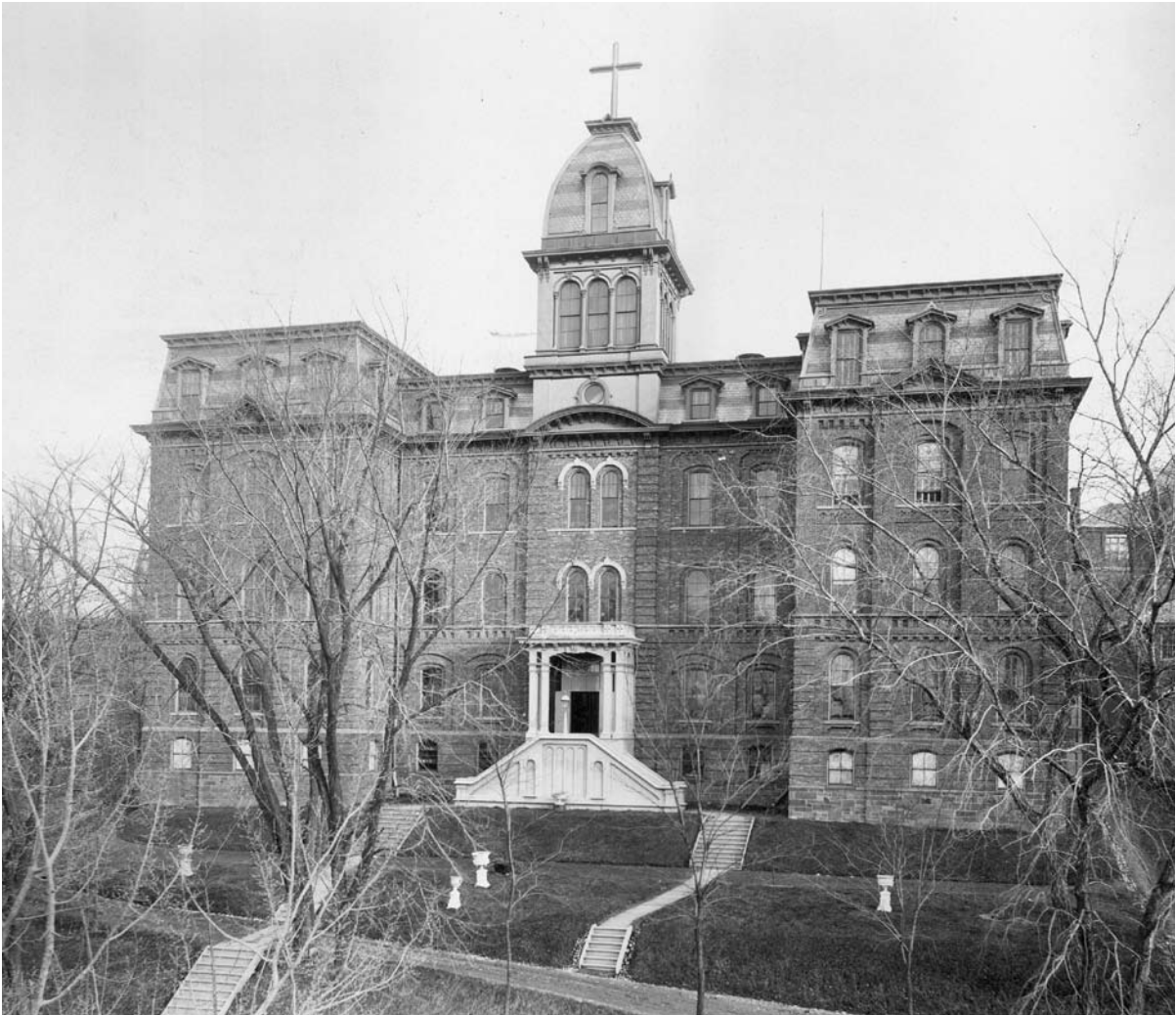
West facade of Troy Hospital on 8th Street. Troy Hospital, Troy, N.Y., 1893. Courtesy of the New York State Library, Manuscripts and Special Collections, Albany, New York.
