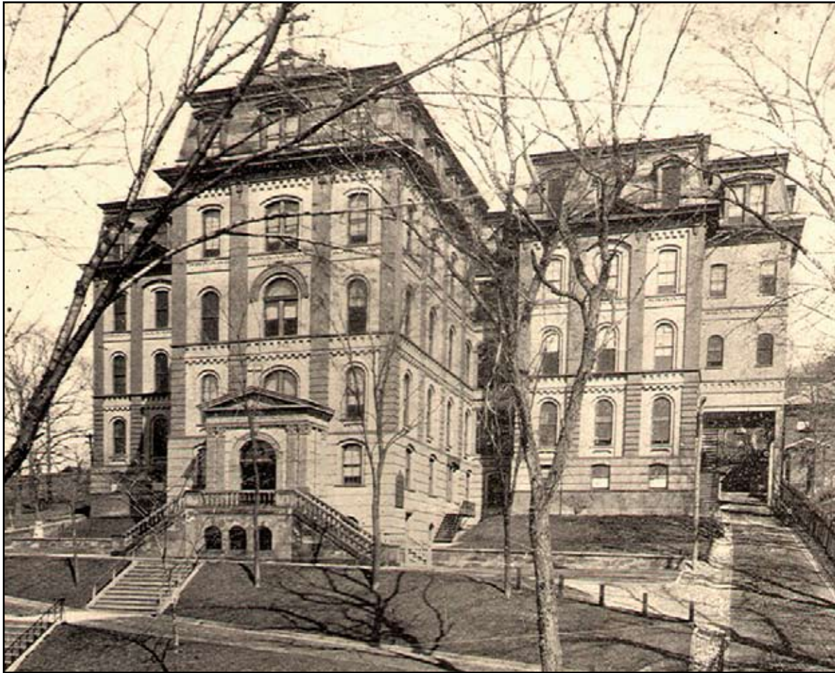
West facade of the Troy hospital, c.1900. Note the south tower, possibly for fire stairs, with a porte-cochere for ambulances. Courtesy of the Daughters of Charity Archives.
