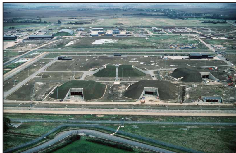
Figure 2. RAF Molesworth in 1987, showing bunkers for ground-launched cruise missiles deployed there briefly that year.
