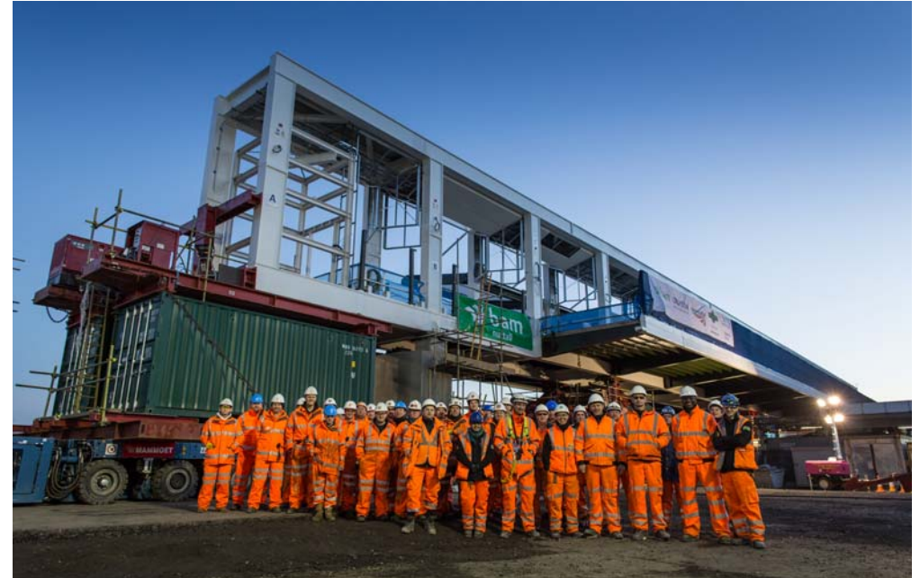
East Croydon Station Footbridge – November 2012.
