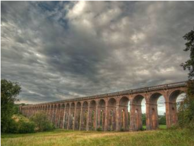
Ouse Valley Viaduct
