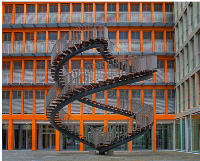
Figure 6. Project of double-spiral sculptural stair case outside KPMG in Munich
