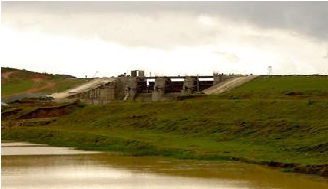
Karapuzha Irrigation Project
