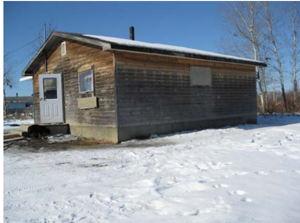
Picture 12. This house in Pikangikum is currently utilized. The owner raised a family with 14 children in this house (March, 2010).
