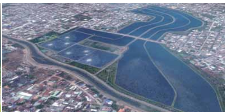
Wastewater treatment plant, 200 000 PE (Ho Chi Minh City, Vietnam)
