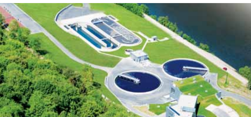
Wastewater treatment plant, 93 100 PE (Namur, Belgium)
