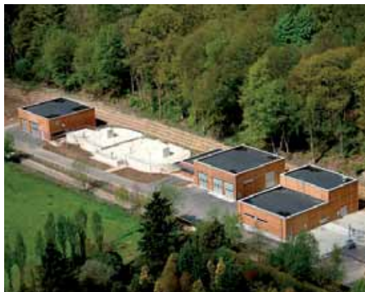
Wastewater treatment plant, 13 000 PE (Louvain-la-Neuve, Belgium)
