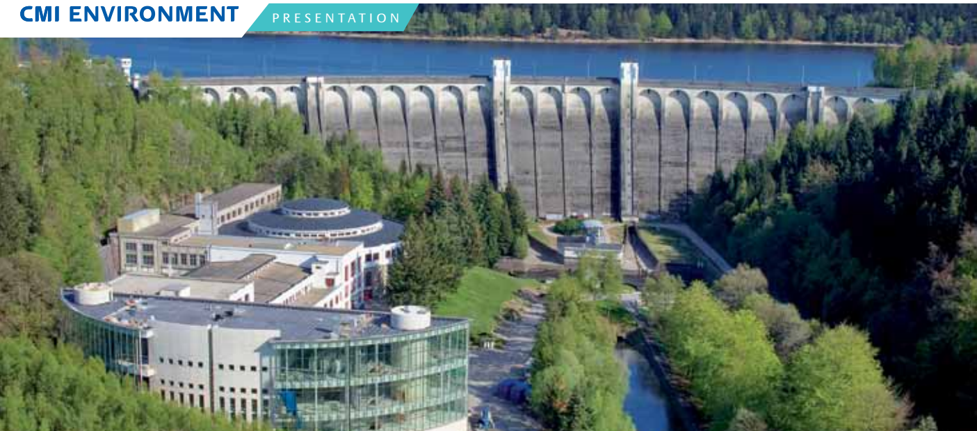
Drinking water treatment plant, 65 000 m 3 /d (Eupen, Belgium)
