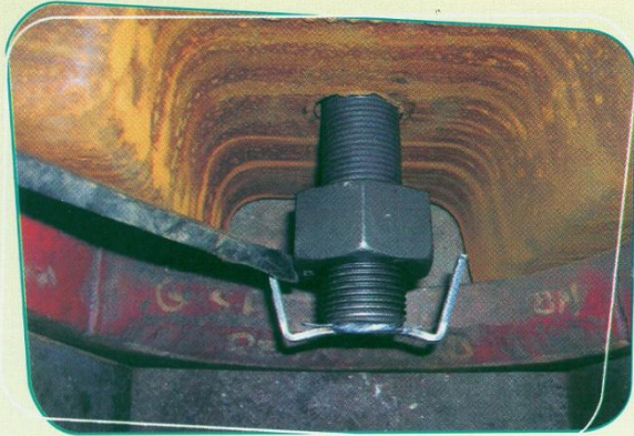
Figure 1 Bend Locking tabs away from nut.
