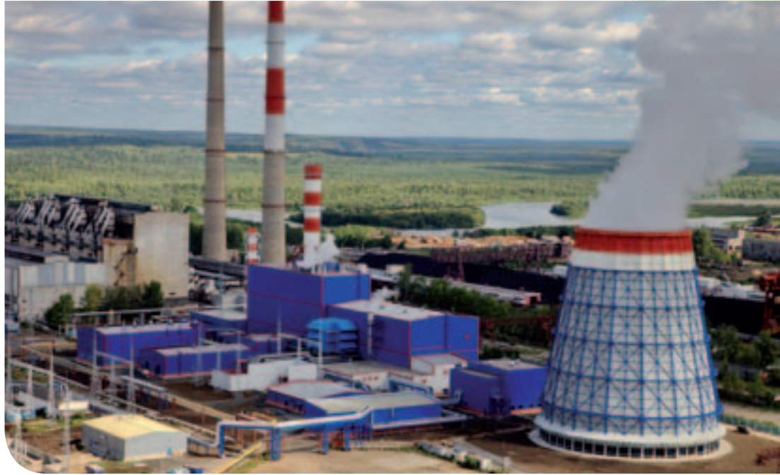
► No faulty performance was observed in the boilers commissioned by CMI Energy in 2011, a demonstration of the quality of the work carried out.
