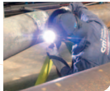
► Pipework welding operations on equipment moved to CMI Services workshops.
