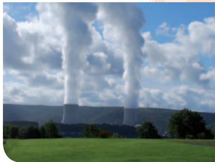
► Whether nuclear power stations are shut-down, dismantled or their life extended, CMI Services, a nuclear safety specialist, will be able to intervene on the facilities for many years to come.
