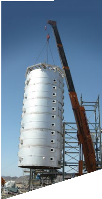
Nesa reactor thermal furnace being unloaded before on-site erection.
