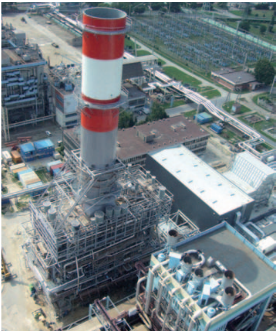
In 2010, CMI Energy confirmed its technological leadership on the market for heat recovery steam generators installed behind combustion turbines in combined cycle power stations.
