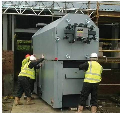
Figure 6.12: Picture of Viessman Pyrotec (740 kW)
