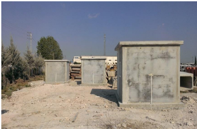
Figure 6.3: Picture of test buildings for demonstration of the novel composite walls in Adana, Turkey
