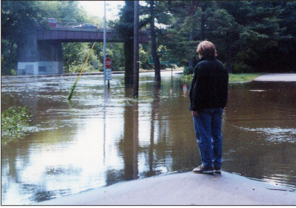
Sawmill River reclaims the Sawmill River Parkway, 1999
