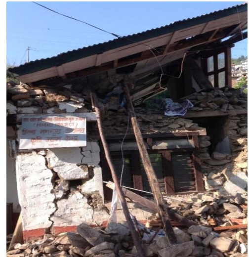
Figure 4: Damaged rural agriculture service centre
